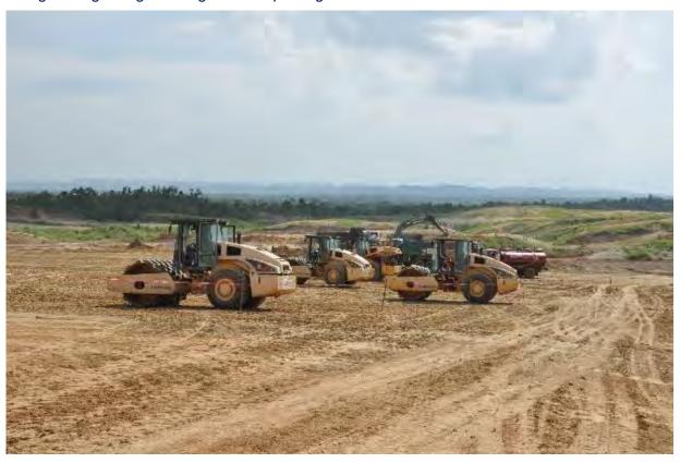
Designated grading levelling and compacting earth surface
