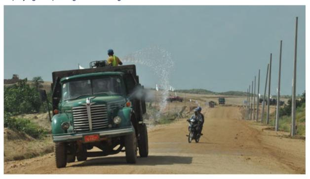
Spraying and pouring water to mitigate dust emission
