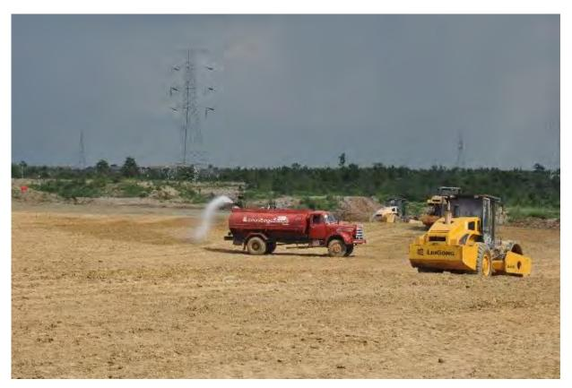
Spraying and pouring water to mitigate dust emission
