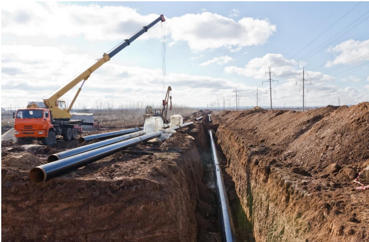
Figure 4.41: Example of Open-Cut Construction Method for Pipeline
