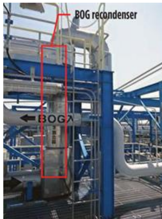
An In-Line BOG Recondenser designed by JFE Engineering Corp.
