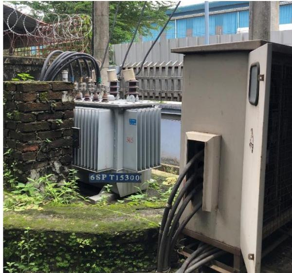
Figure 3-17 Photo of 315 KVA Transformer
