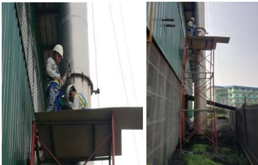
Figure 4.3 Photos of Boiler Stack Gas Monitoring
