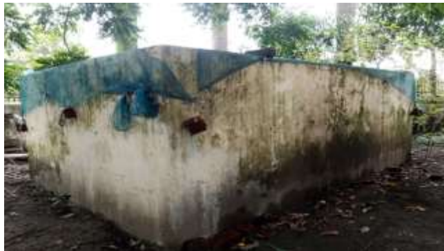
Figure 3.30 Water storage tank for Firefighting
