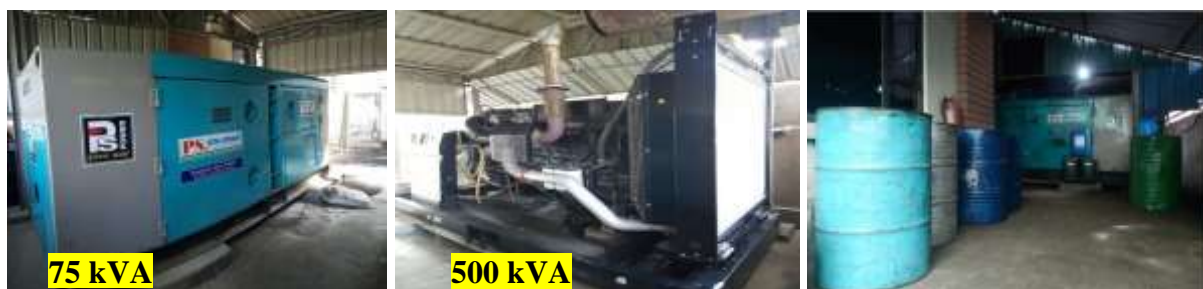
Figure 3.17 Generators and Diesel Storage
