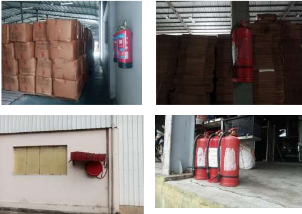
Figure 3.29 Fire Extinguisher and firefighting Equipment (Thai Faster Products and M.K Co., Ltd)
