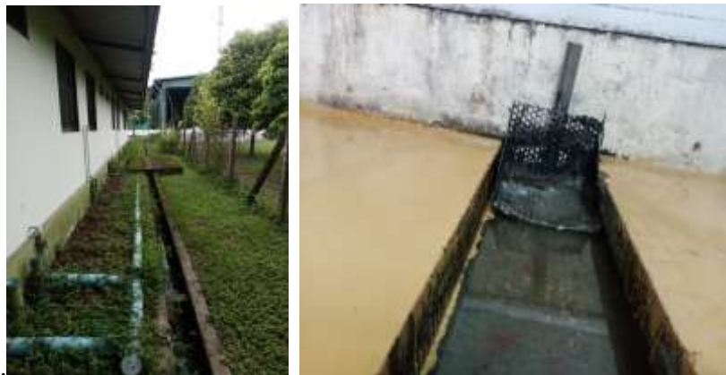
Figure 3.25 Photos of Drainage system
