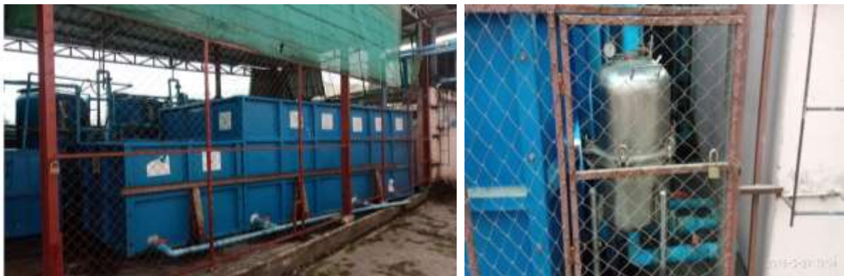
Figure 3.19 Water Treatment System
