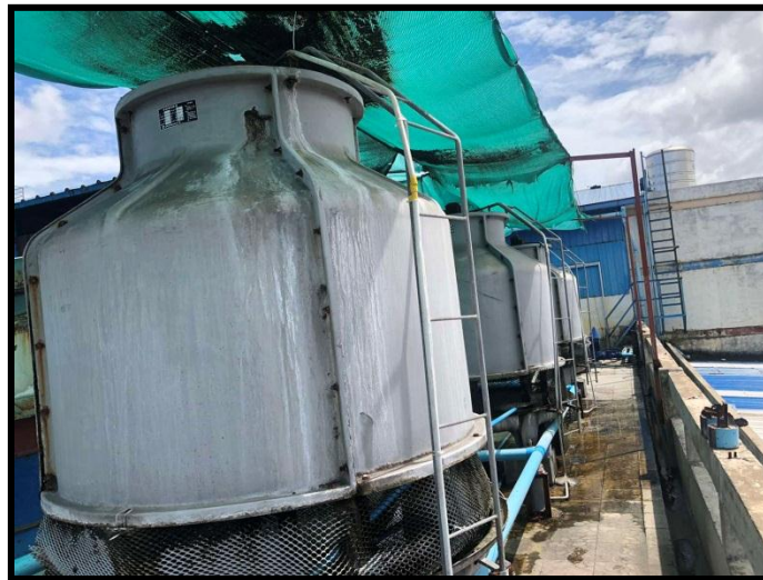
Figure 3.12 Photo of Water Tank
