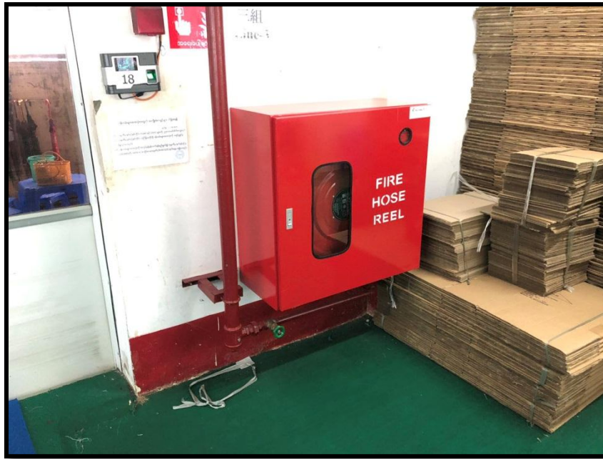
Figure 7.2 Photos of Facilities for Fire prevention and Safety Signboards
