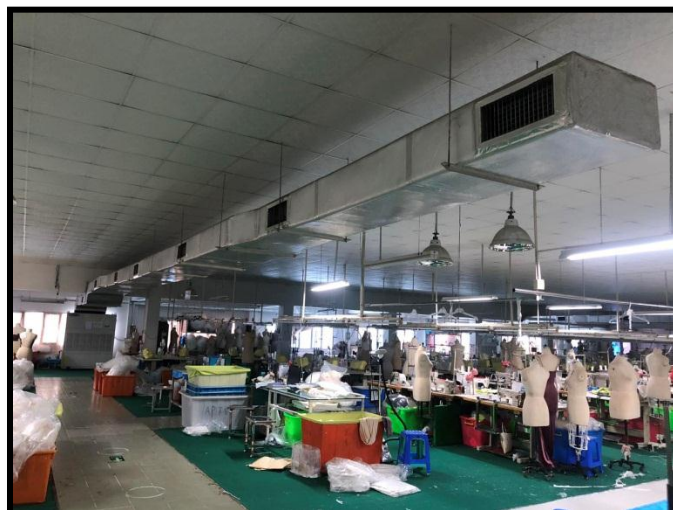
Figure 3.15 Photo of Ventilation
