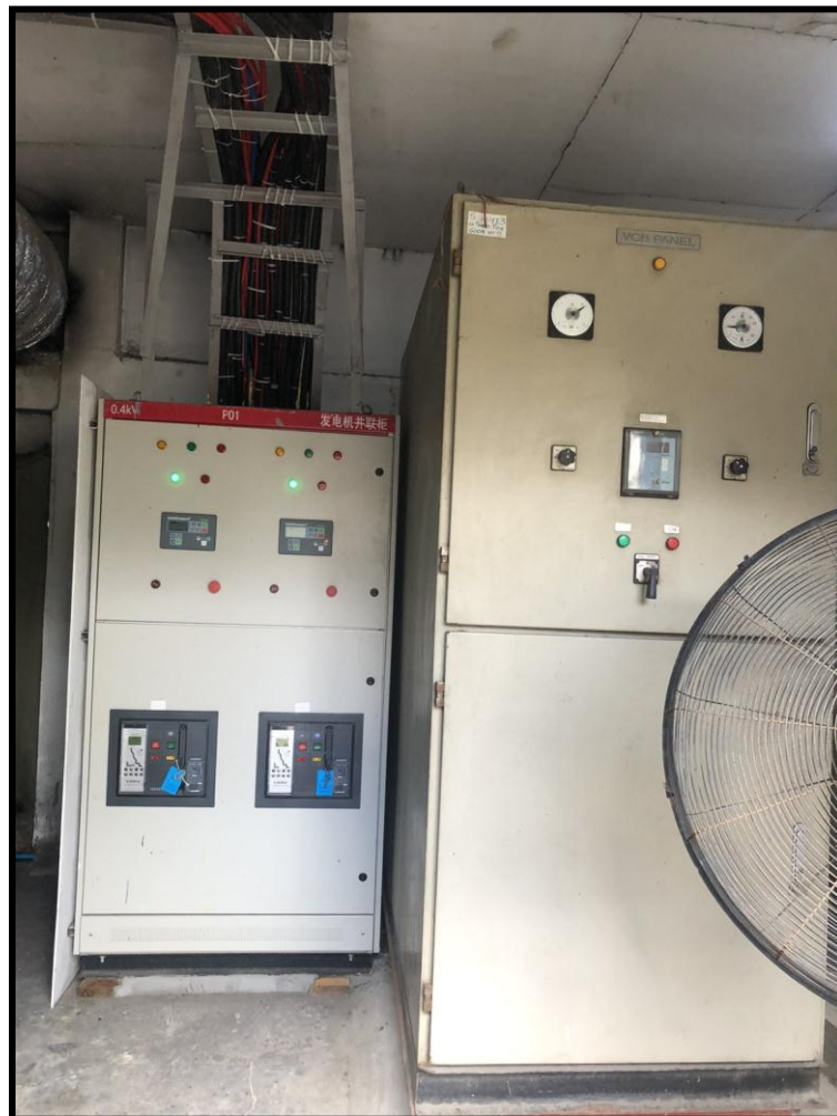
Figure 3.11 Photo of Generator
