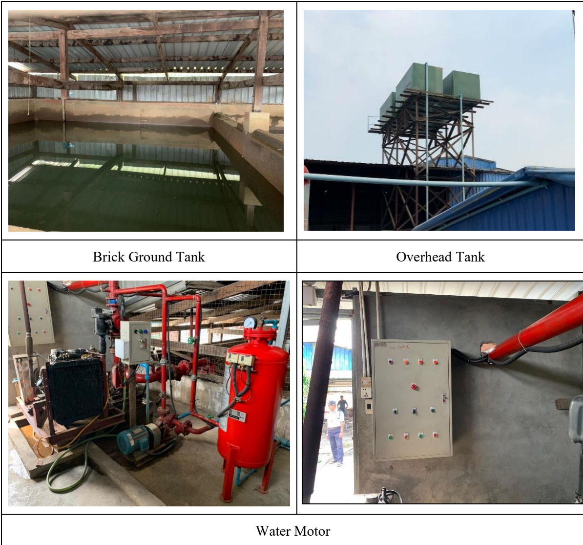
Figure 2-18 Water Recharge System
