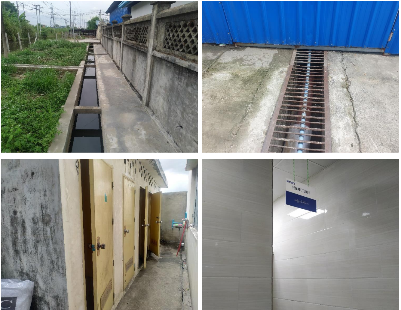
Figure 3-14 Drainage and Toilet facility
