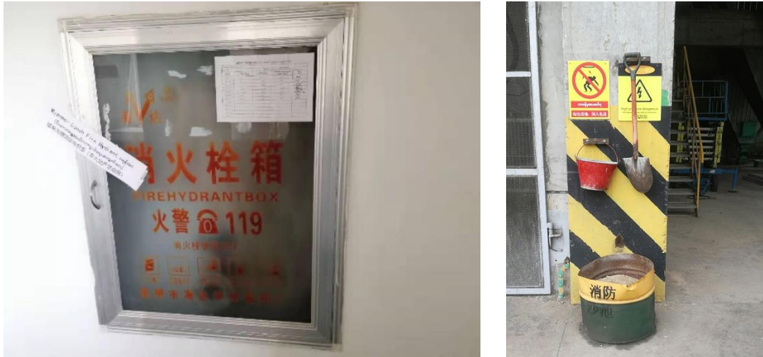
Figure 6-15 Fire Hydrant and Equipment
