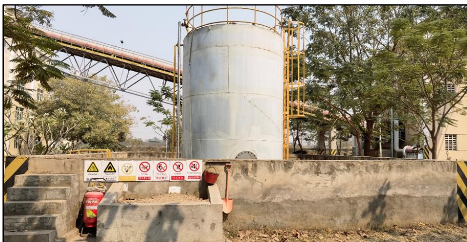
Figure 6-8 Fuel Storage Tank
