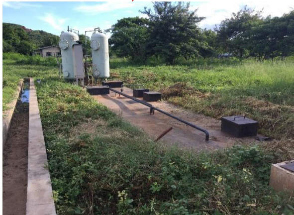
Figure 3-18 Domestic wastewater treatment system
