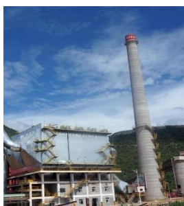
Electrostatic Precipitator (EP)
