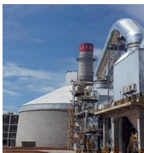
Electrostatic Precipitator (EP)
