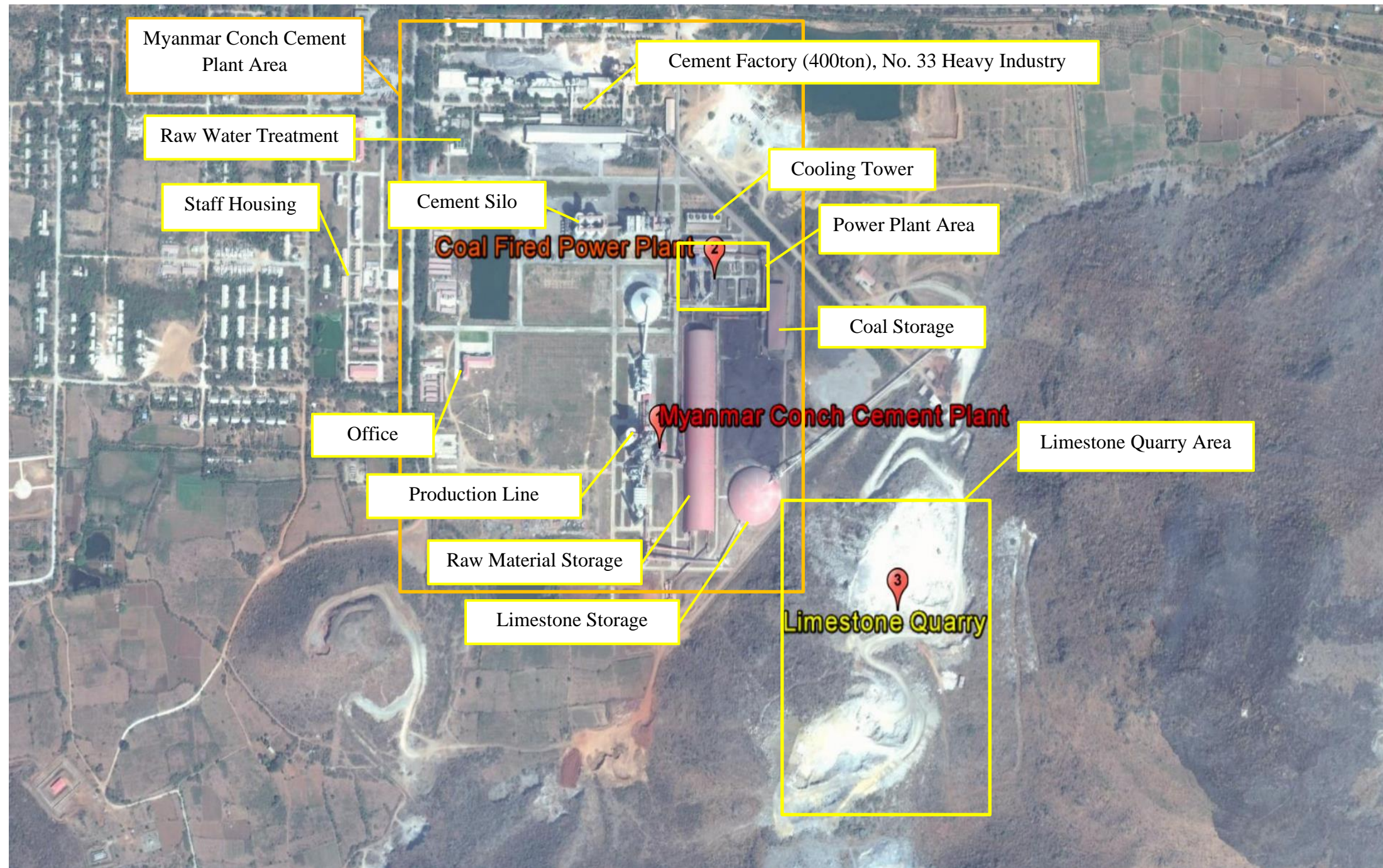
Figure 3-3 Myanmar Conch Cement Plant and associate facilities including Captive Power Plant and Limestone Quarry
