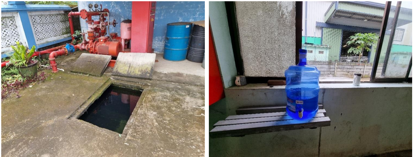
Figure 3-7 Water storage and drinking water supply
