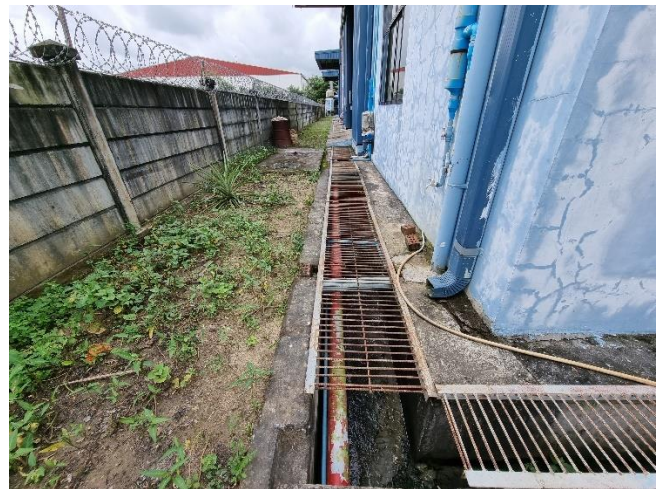
Figure 3-10 Drainage System of Factory
