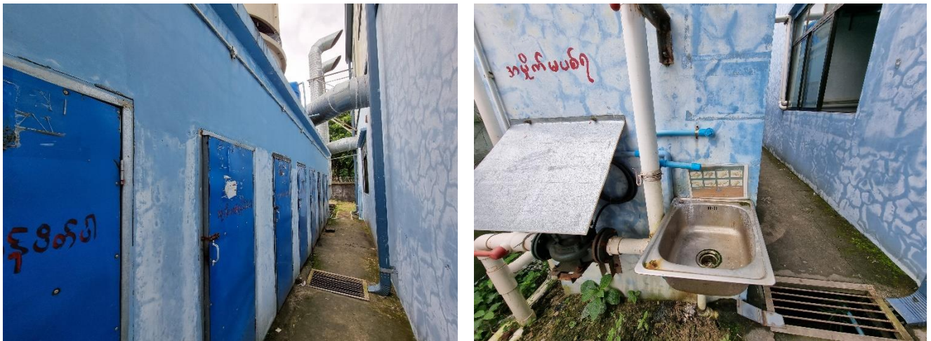
Figure 3-13 Toilet Facilities Photos
