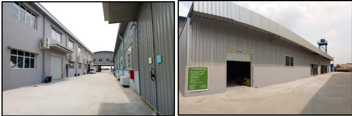
Warehouse and Recycle Room, Disposal Room
