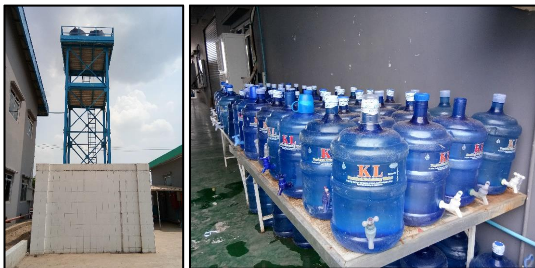
Figure 1-30 Water Tanks and Purified Drinking Water Bottles
