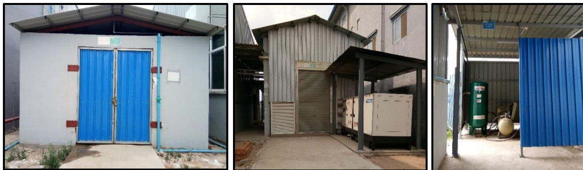
Two Boiler Rooms, Generator Location and Compressor Room
