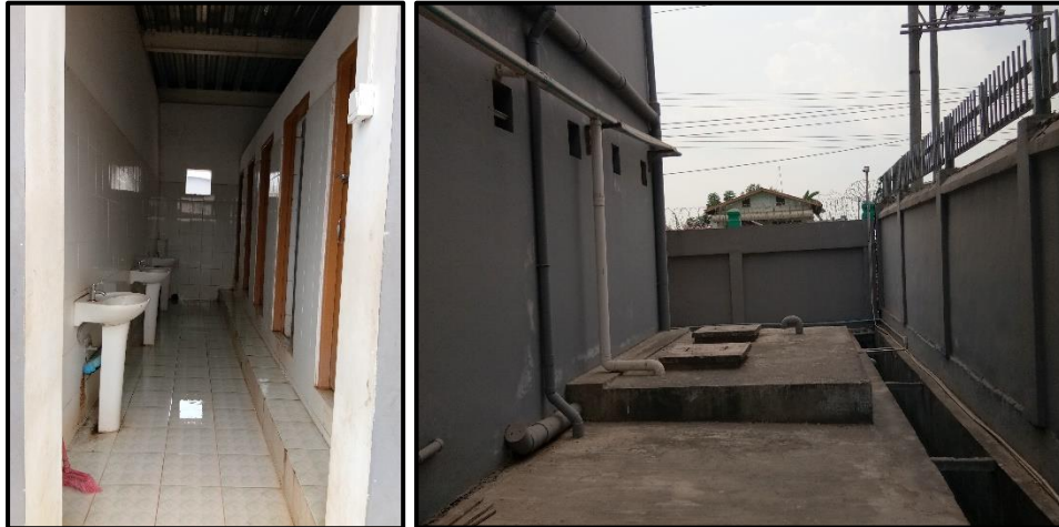
Figure 1-32 Toilets, Septic Tank and Drainage
