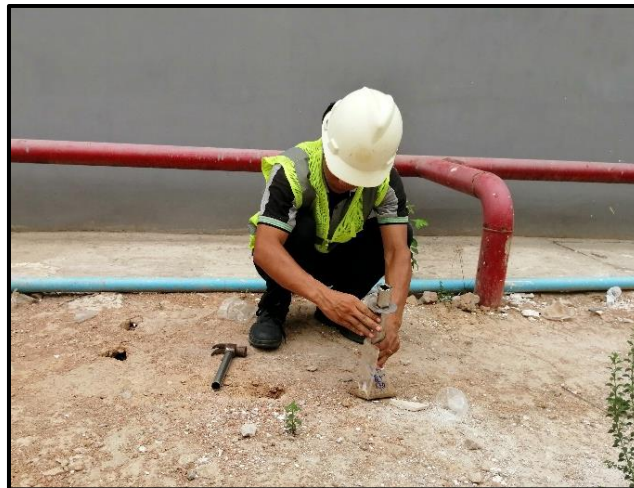
Figure 5-13 Soil Sample Taking in The Project Site (ID 1)
