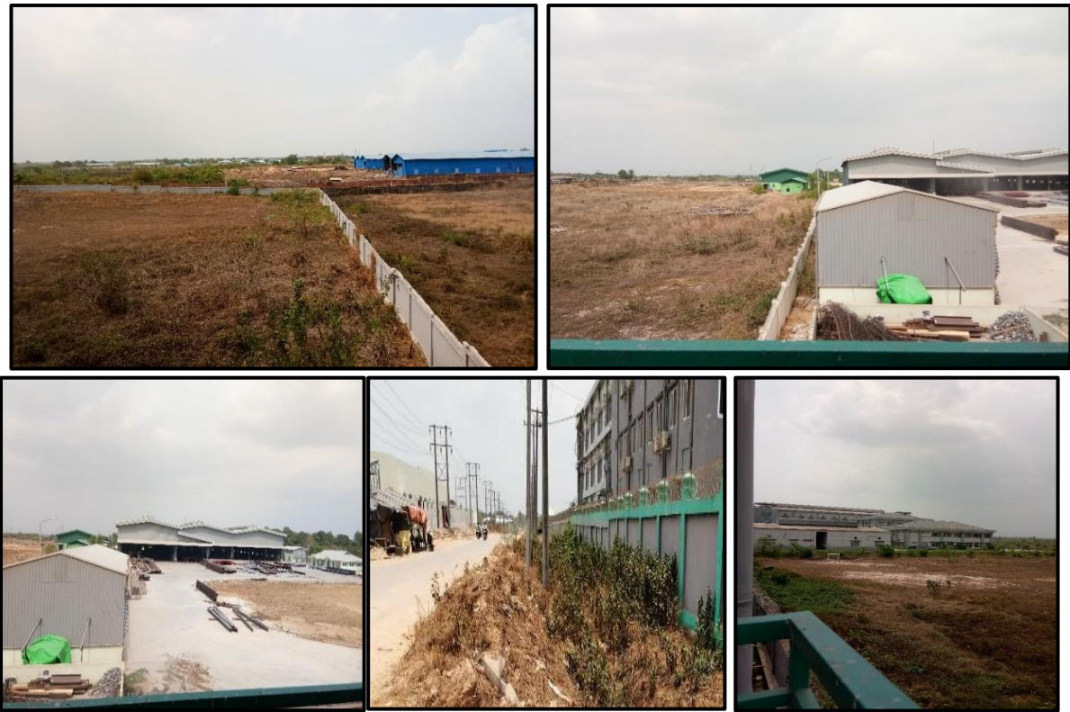
Figure 5-18 Visual Component around Project Site
