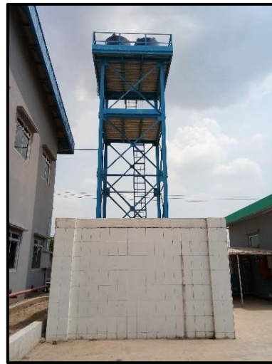
Figure 9-7 Fire-fighting Water Storage Tank
