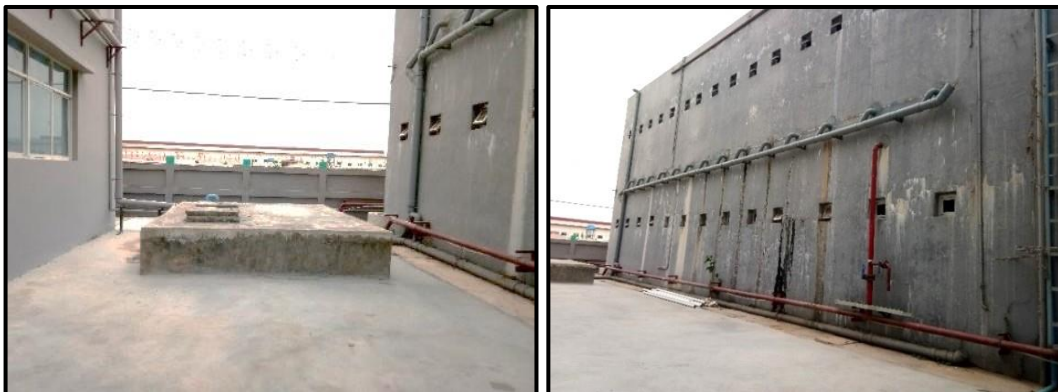
Figure 9-1 Sewage System with Septic Tank
