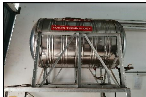
Figure 9-4 Diesel Storage Tank
