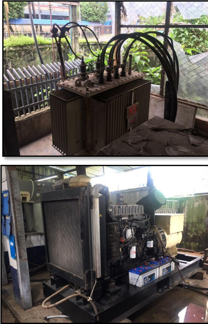
Figure 3-12 Photos of Transformer and Generator
