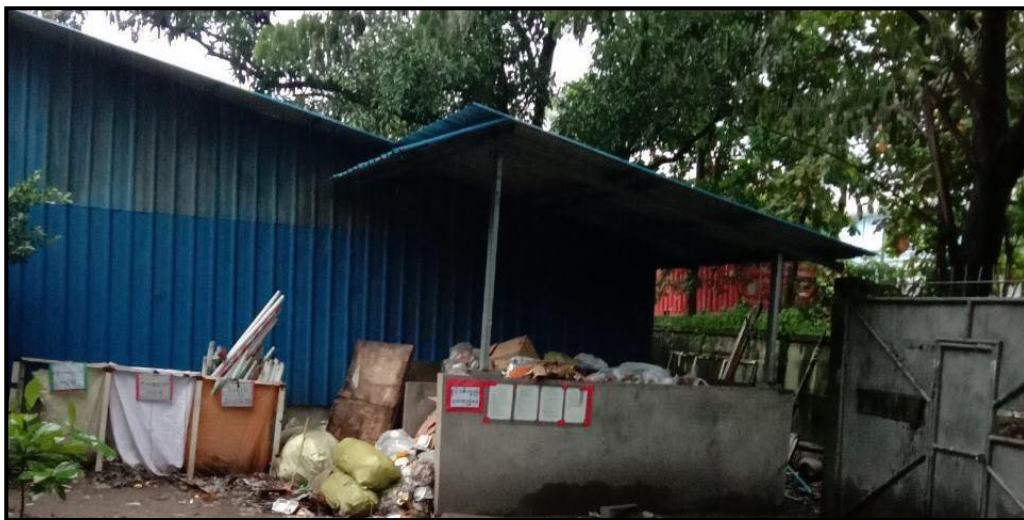
Figure 3-16 Photos of Garbage Room
