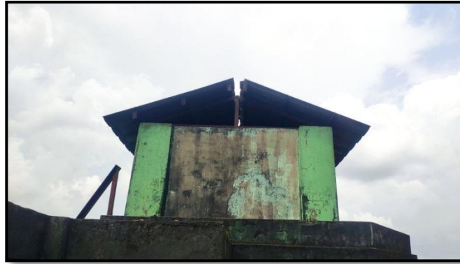
Figure 3-13 Photos of Water Supply
