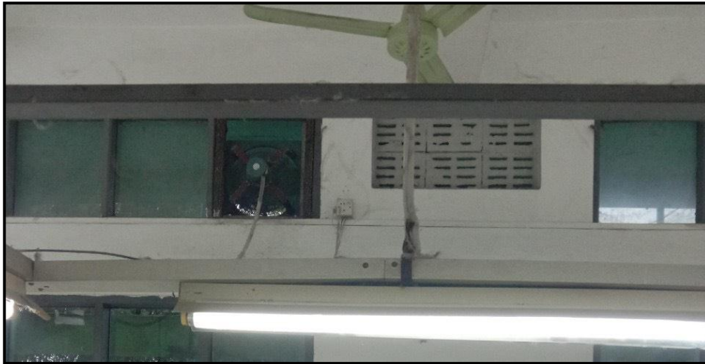
Figure 3-17 Photos of Ventilation
