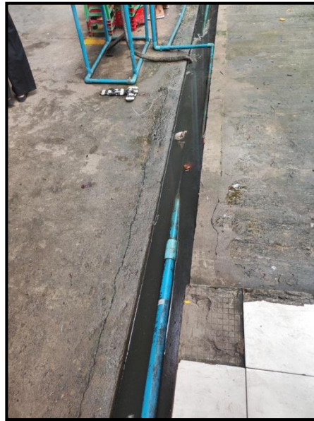
Figure 3-15 Photos of Drainage System
