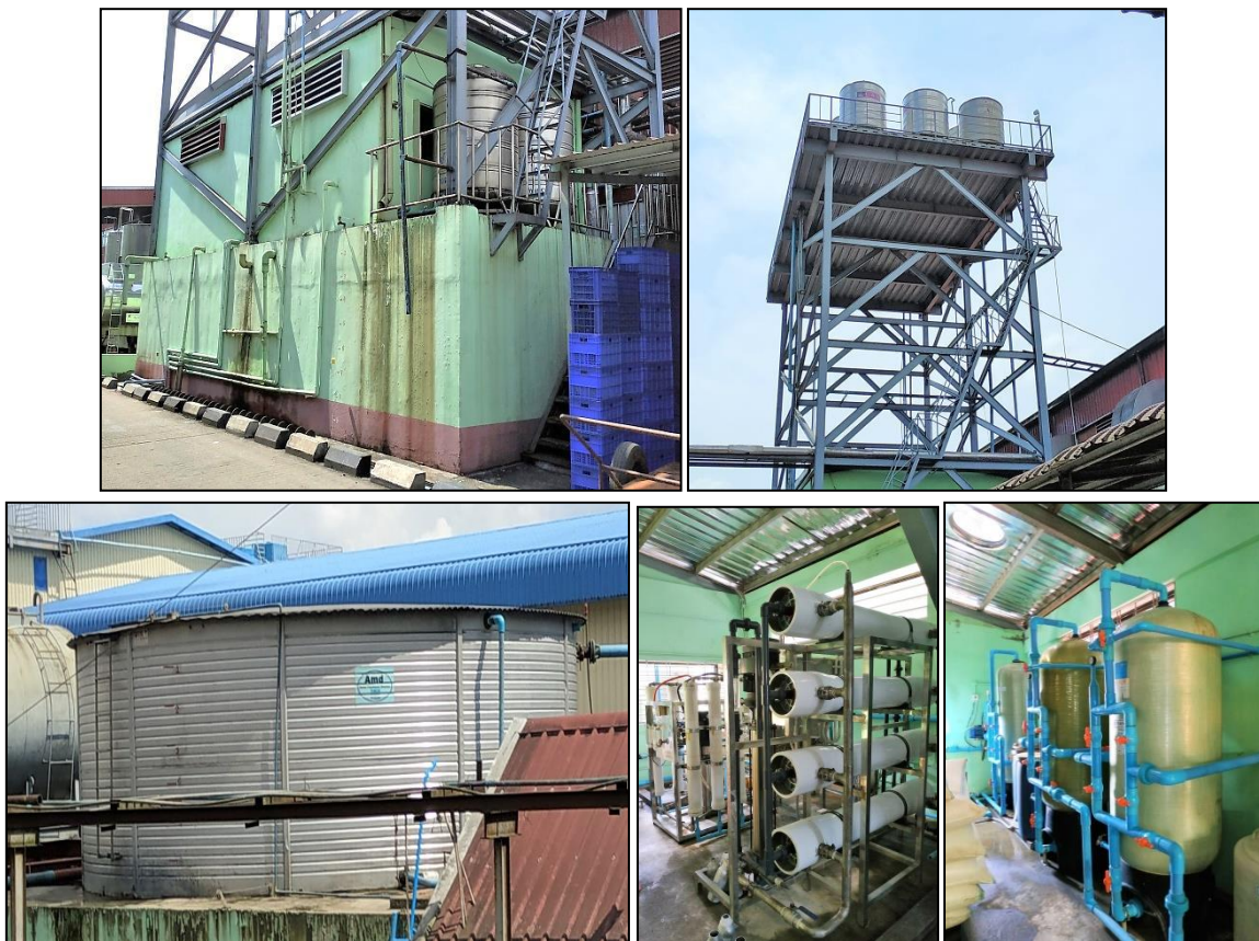
Figure 5.15 Water Storage Tank, Overhead Tank and Water Treatment System
