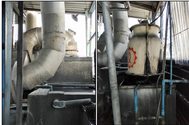
Figure 5.20 Wet Scrubber System for Boiler
