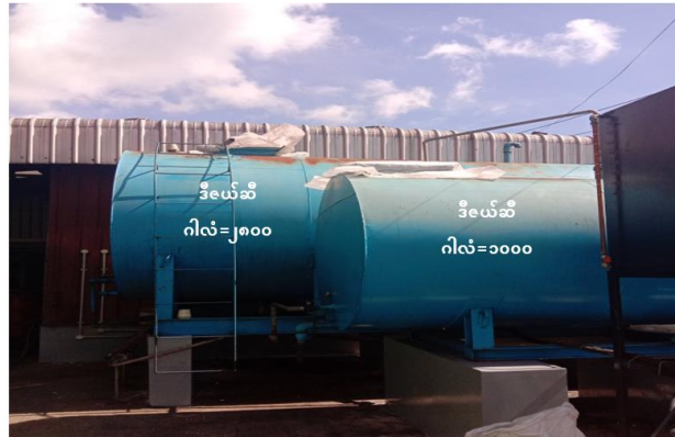
Photos of Diesel Storage Tanks
