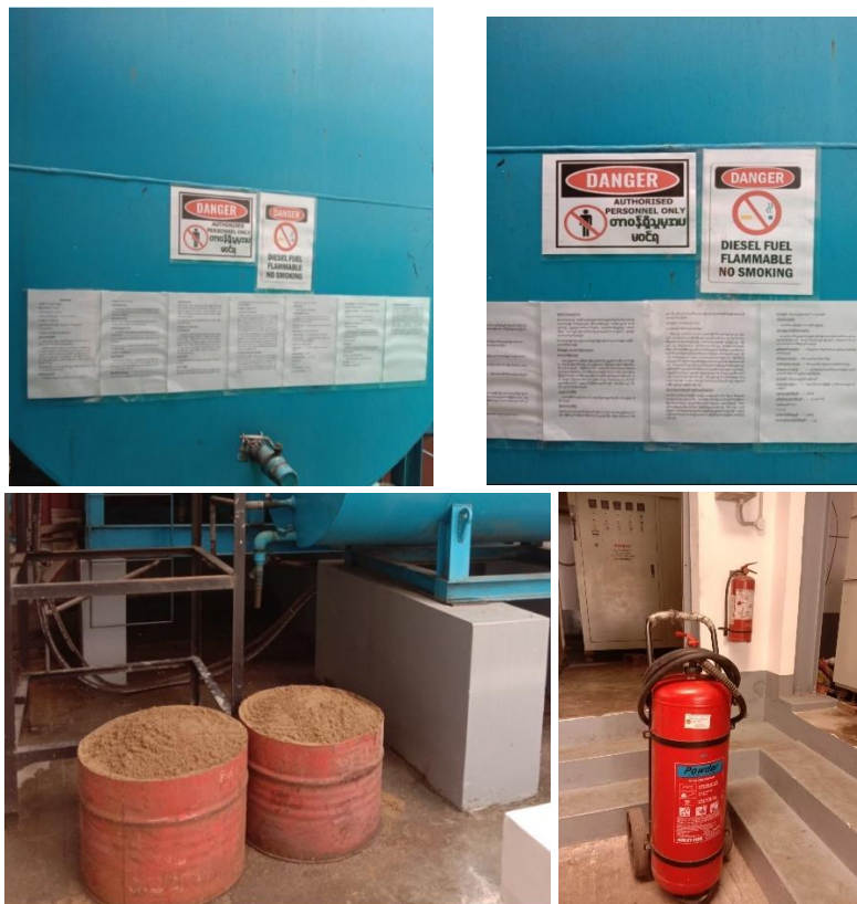
Diesel Storage Tanks with Preventing Unauthorized Person, No Smoking, Caution Sign, MSDS, keeping Sand Tanks and Extinguishers
