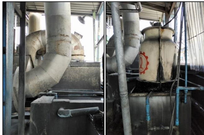
Wet Scrubber System for Boiler
