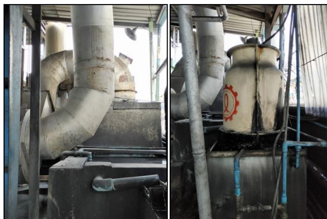
Figure 7.3 Wet Scrubber System for Boiler
