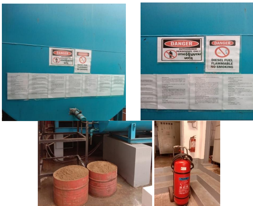
Figure 5.18 Diesel Storage Tanks with Preventing Unauthorized Person, No Smoking, Caution Sign, MSDS, keeping Sand Tanks and Extinguishers
