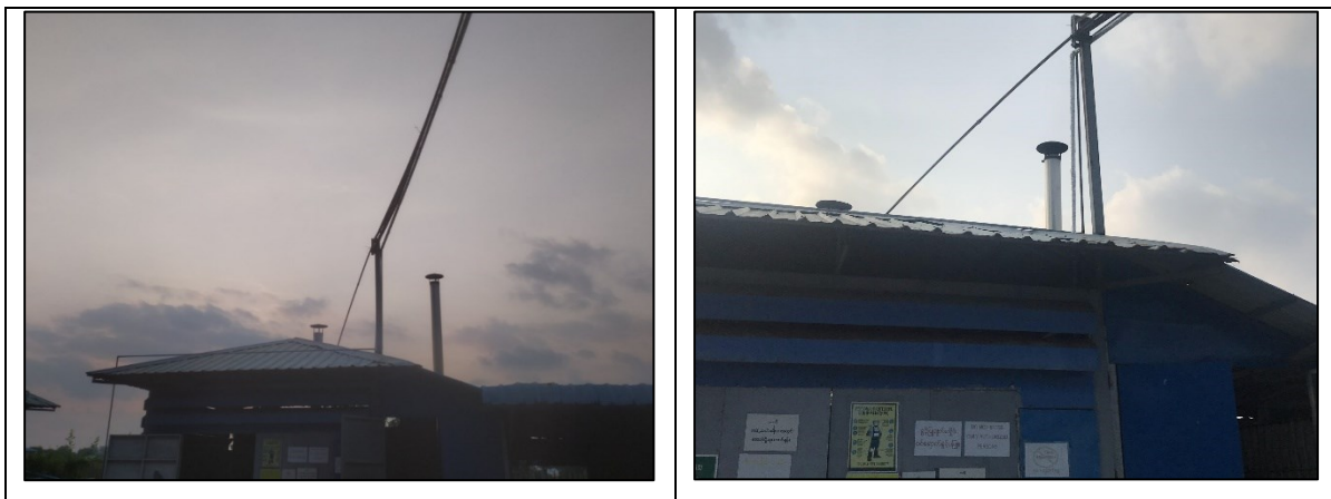
Figure 2-30 Boiler Funnel of Hakers Enterprise Factory
