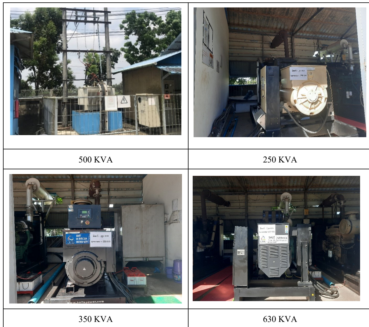
Figure 2-16 Electric Supply Systems of Hakers Enterprise Factory
