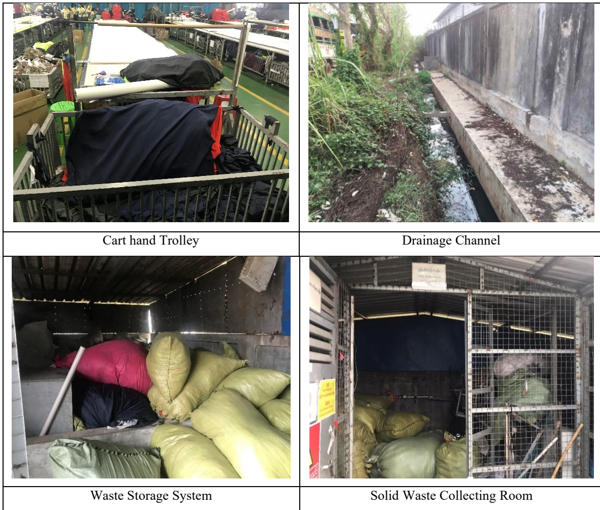
Figure 2-21 Sanitary Facilities of Hakers Enterprise Factory
