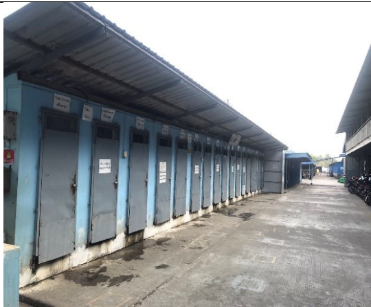
Toilet for Workers
