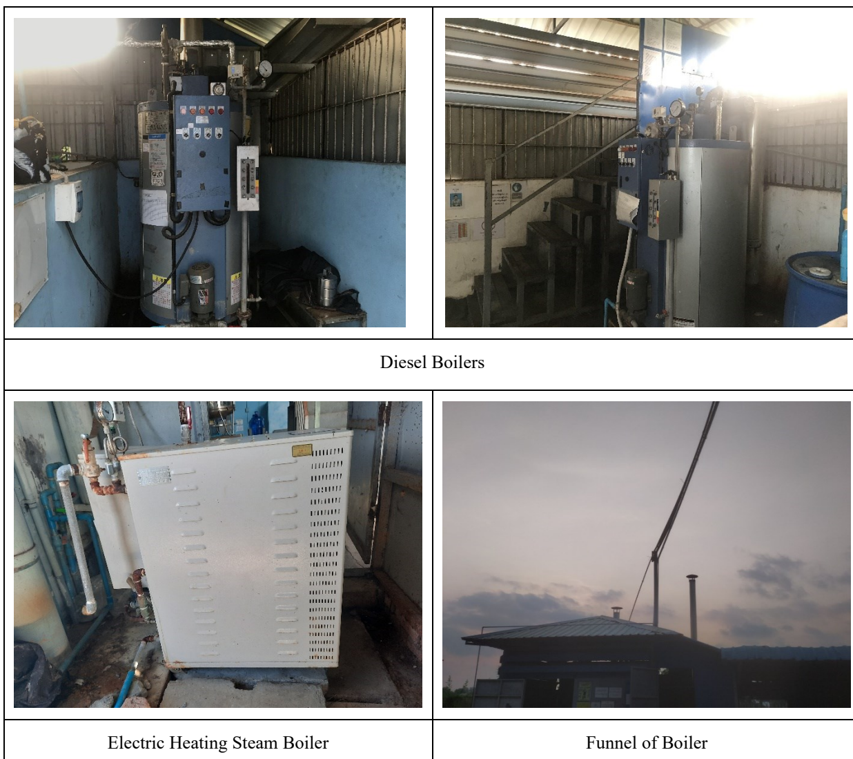
Figure 2-17 Boiler System of Hakers Enterprise Factory
