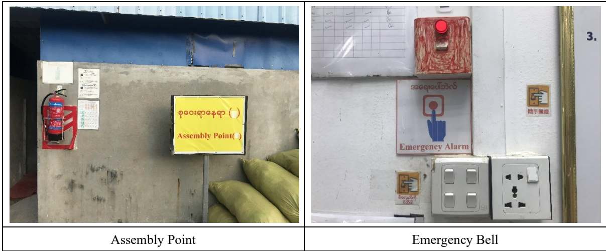
Figure 7-10 Fire Fighting and Emergency Response Facilities at Hakers Garment
