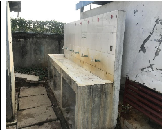
Hand Wash Basin near Toilets
