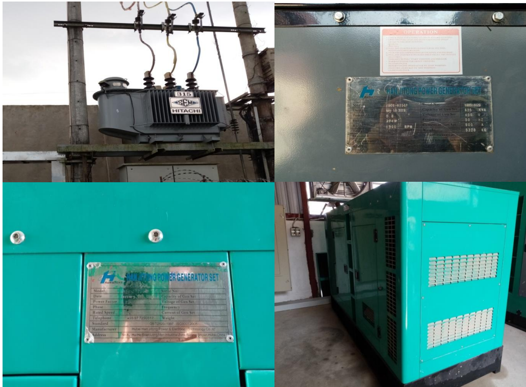
Figure 8 Transformer and Diesel Generator
