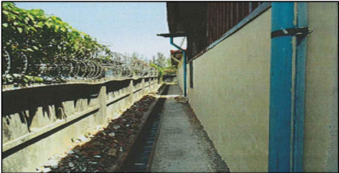
Figure 11 Drain and downpipe condition at Factory
