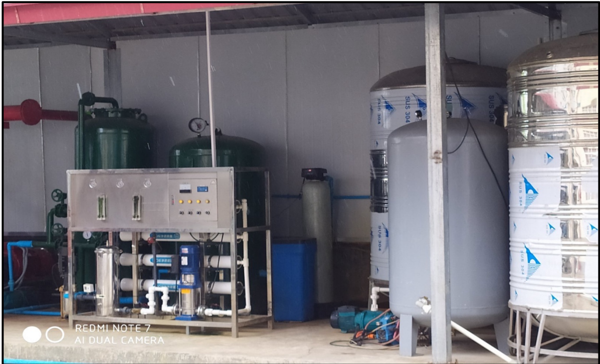
Figure 7 Yacheng RO Water Treatment Plant on site
