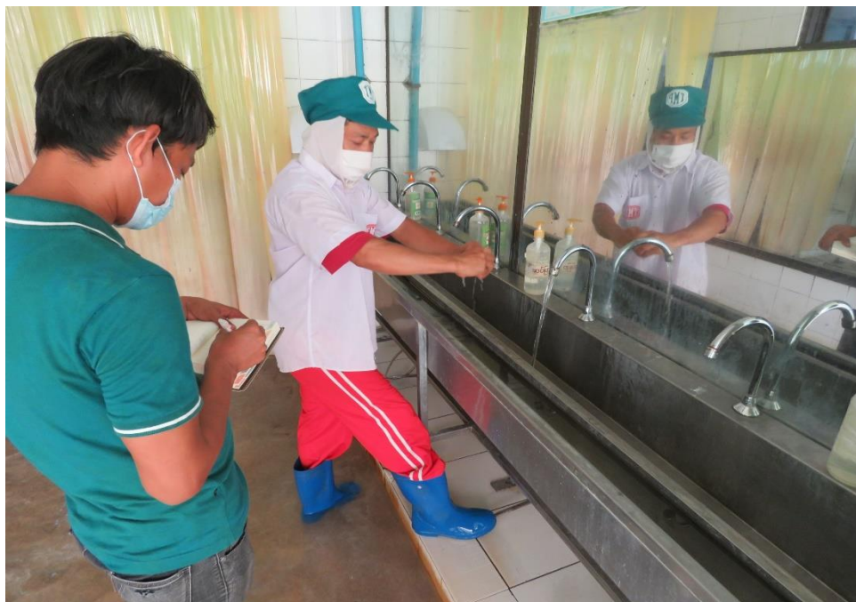
Figure 4.21: Sufficient hand and foot washing facilities (Chlorine level for hand washing is 10ppm and foot dip is 100ppm) at the entrance of the processing area
