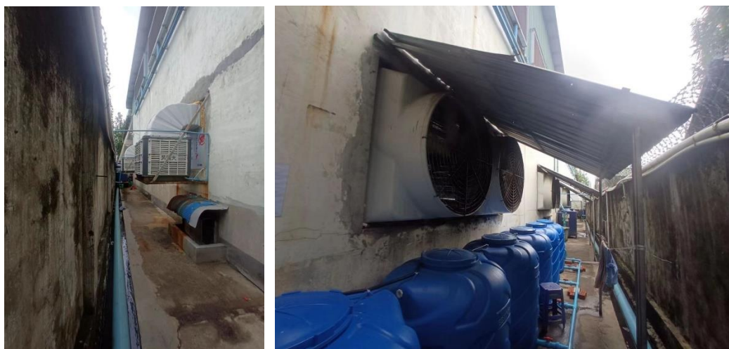
Figure 12. Installed Exhausted Fans for Indoor Factory Air Cleaning
