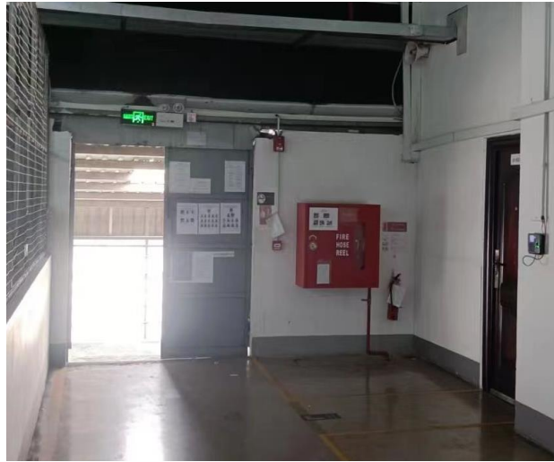
Figure 29. Emergency exits sign are installed
