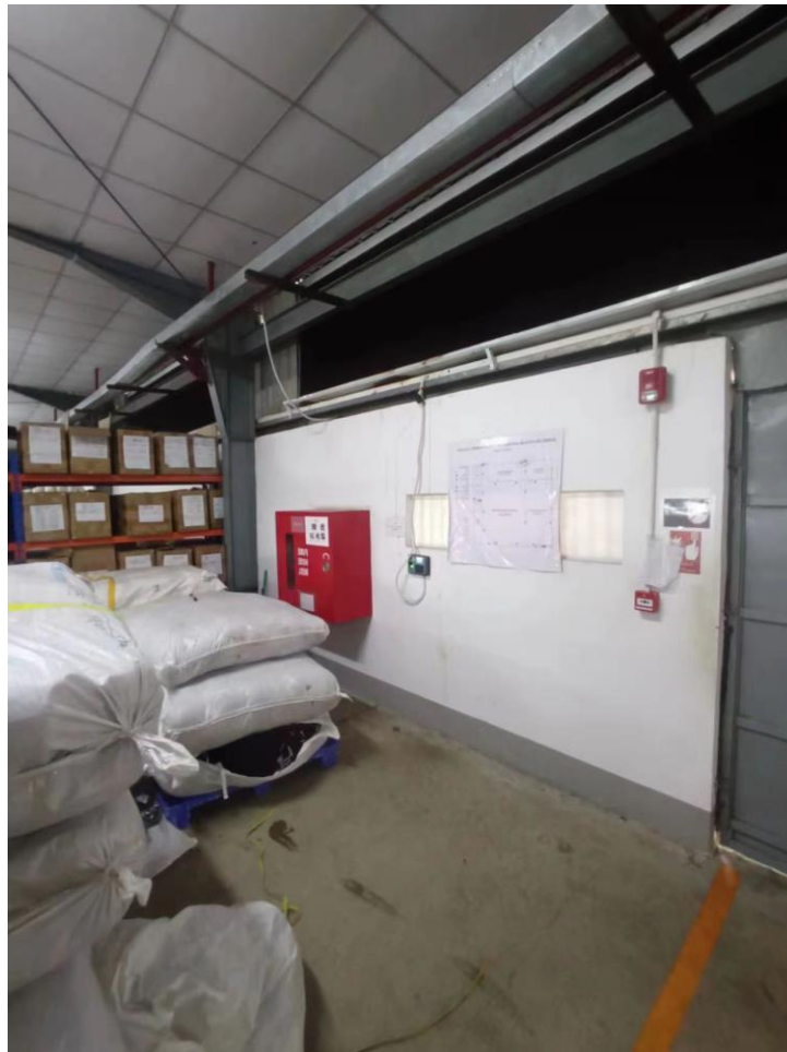
Figure 30. Fire Hose Cabinets and Fire Alarm Is Provided for Emergency Cases
