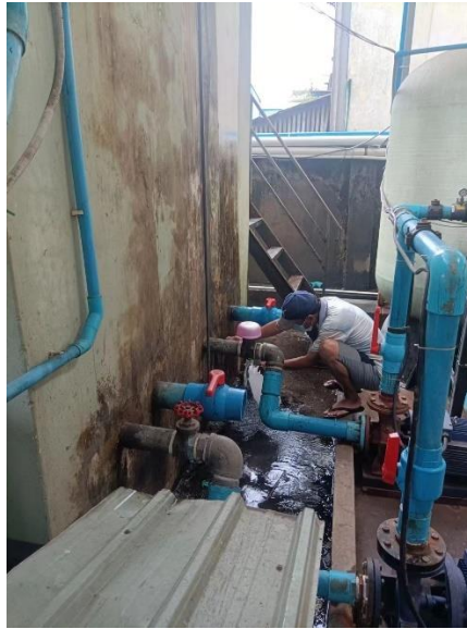
Figure 8. Water Collection from Tube Well Water Concret pool (Concret pool)
