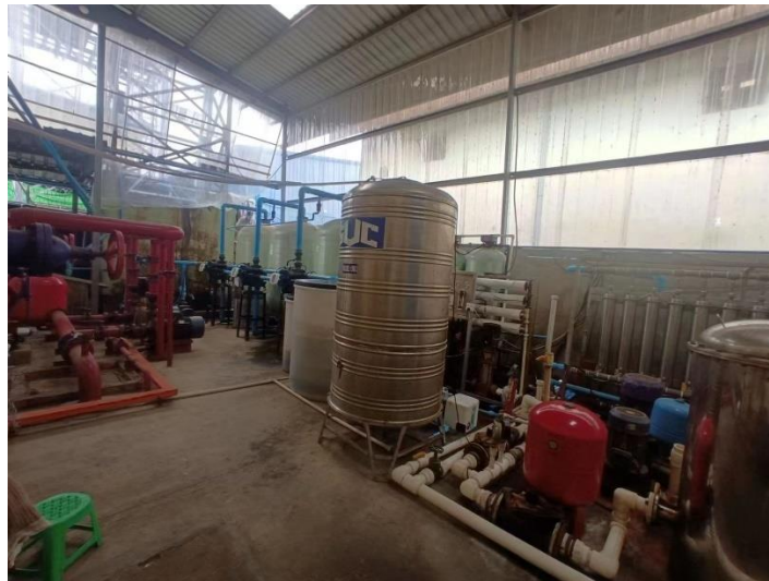
Figure 9. Drinking Water treatment system was installed for labor
