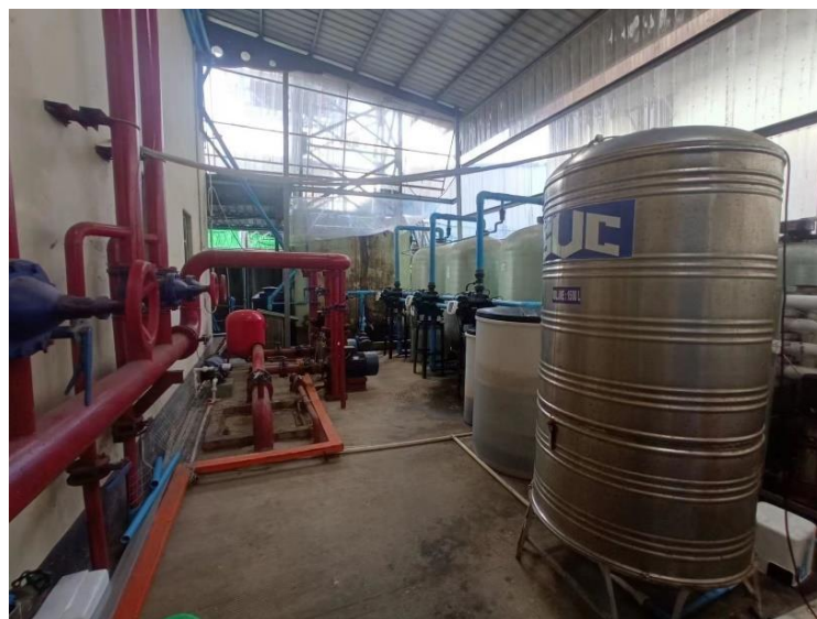
Figure 31. Constructed firefighting unit with high pressure pump
