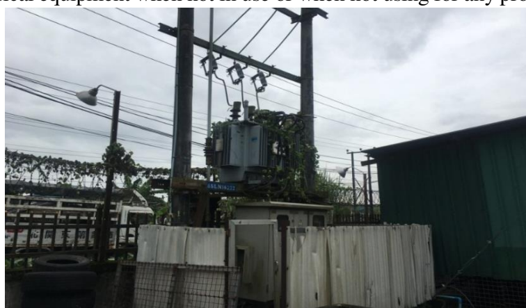
Figure 3-12 Photo of 315 KVA Transformer
