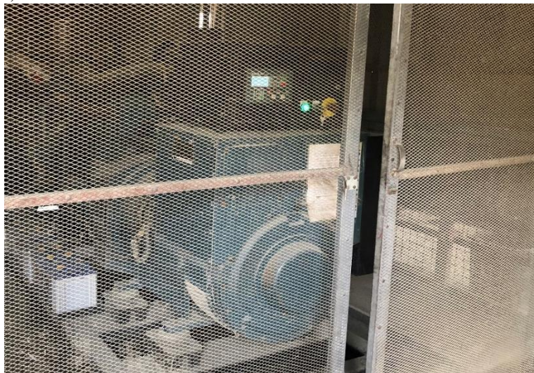
Figure 3-13 Photo of 300 KVA Generator
