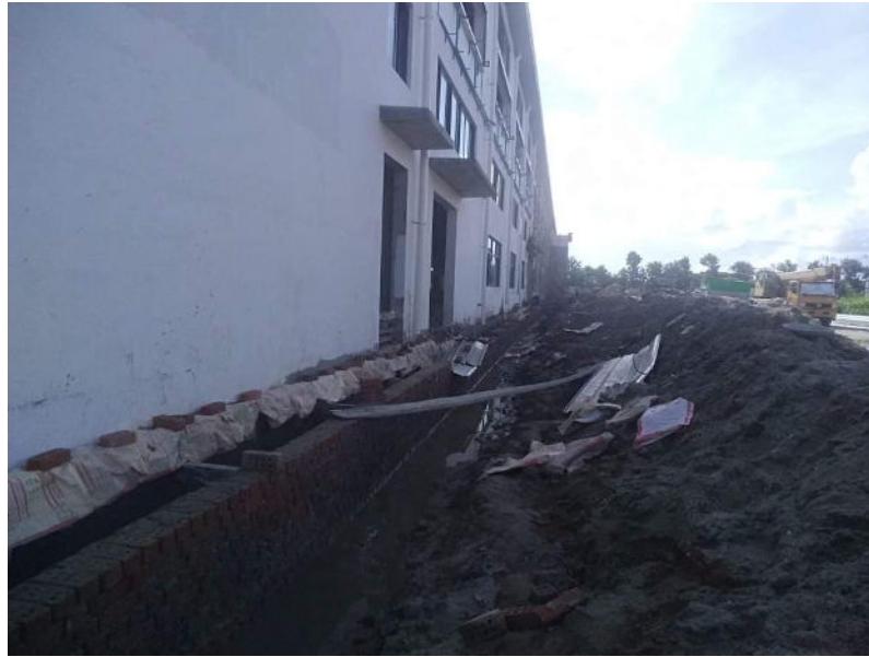
Figure 4.6 - Drainage Channel in the Factory Compound (during construction)
