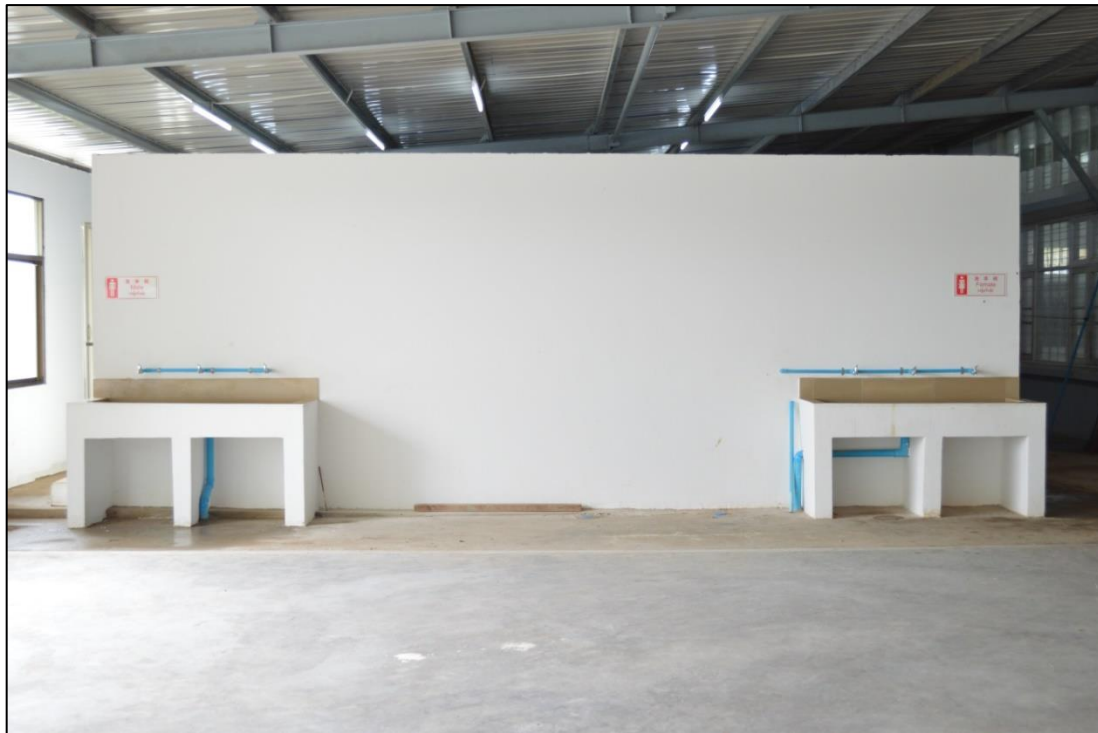
Figure 2-18 Toilets for Factory Employees
