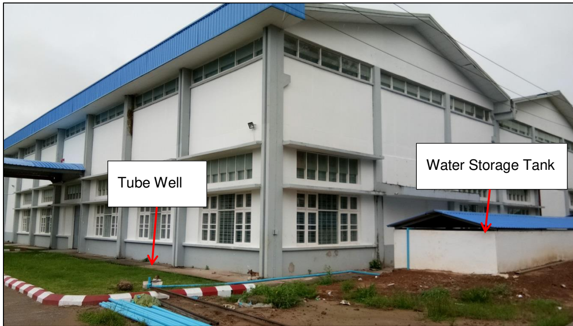
Figure 2-12 Water Storage Tank
