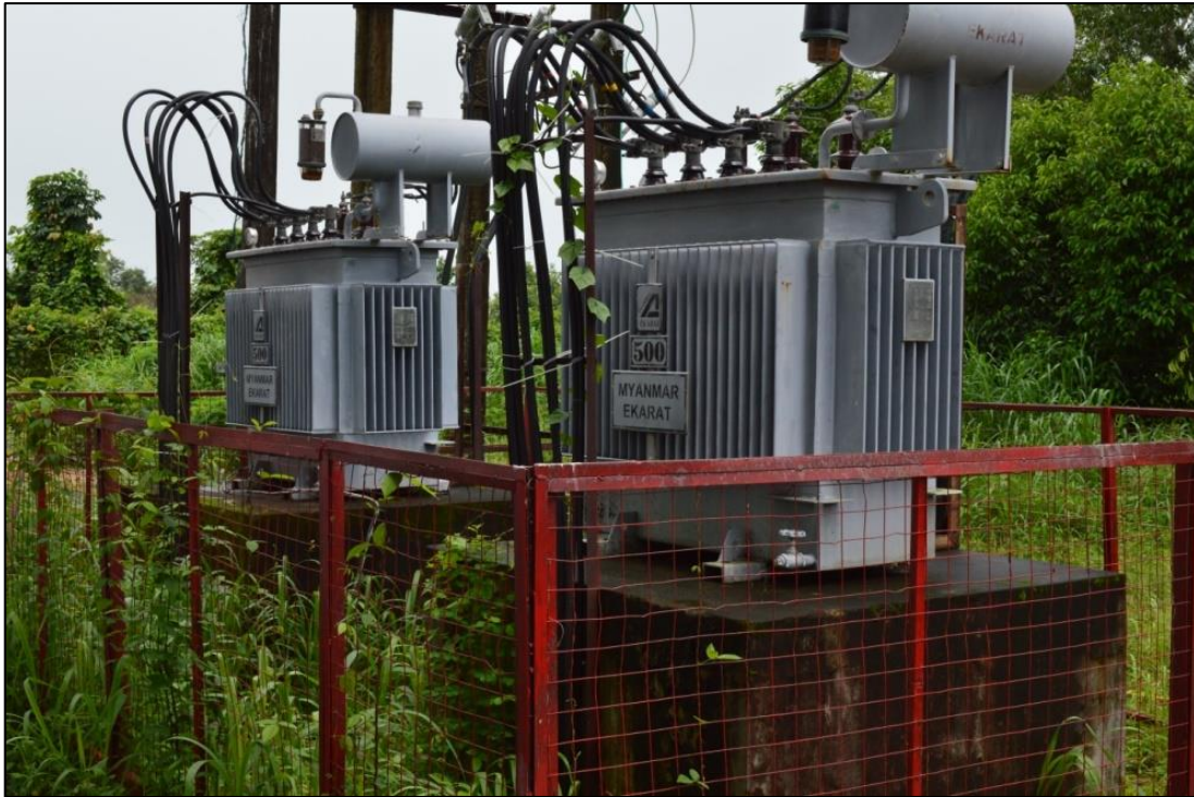
Figure 2-15 One is Amity Transformer and Another One is MEC Transformer
