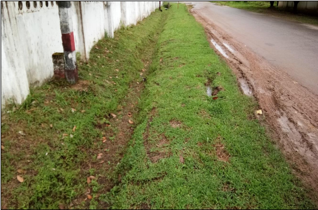
Figure 4-6 Indagaw Industrial Drainage Network
