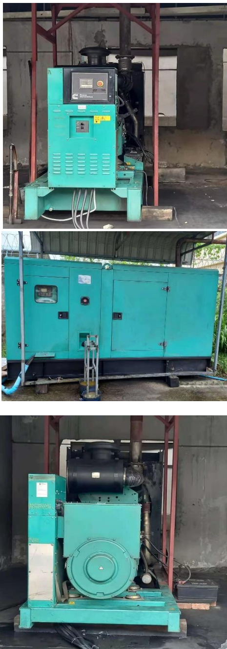
Figure 3-22 Photos of 690 KVA, 440 KVA & 150 KVA Generator
