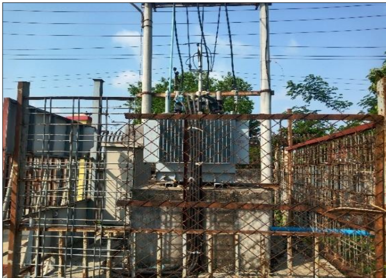
Figure 3-21 400 KVA Transformer
