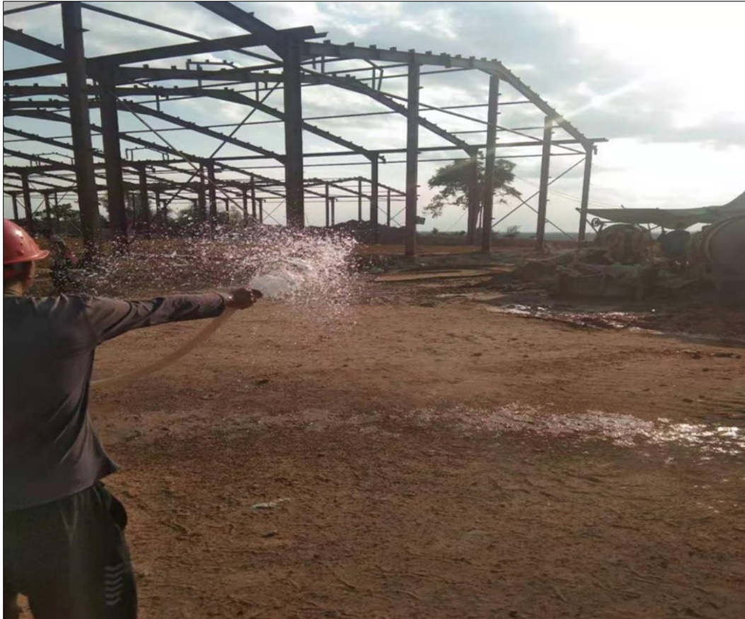
Figure 5-2 Water spraying system in the project area
