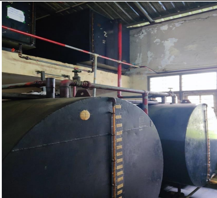
Figure 4.7 Diesel Storage Tank
