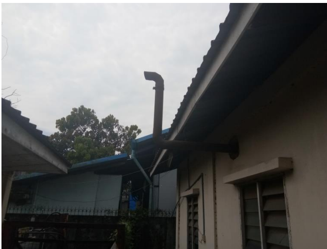
Chimney for Generator
