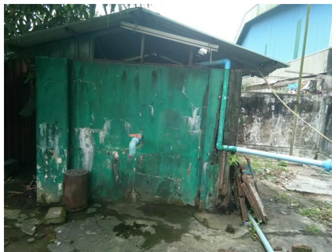
Ground Tank for Firefighting
