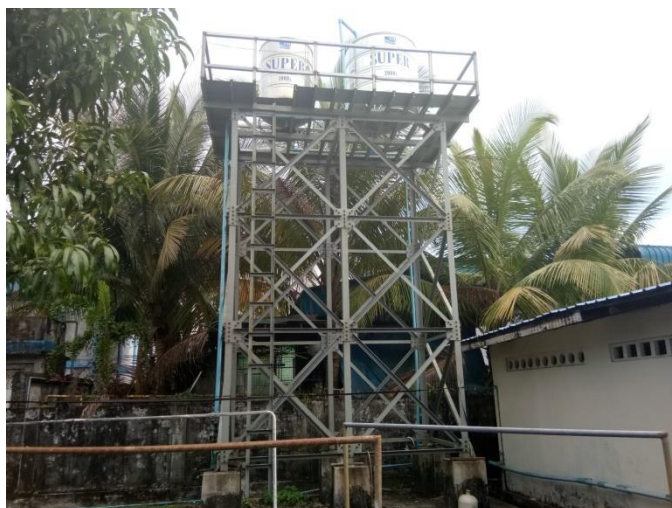
3,000 Gallons Overhead tank
