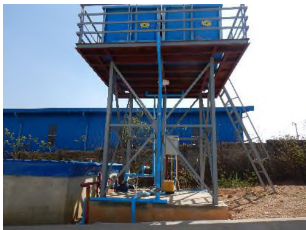
Figure 17: Water Storage Tanks and Fire water Tank
