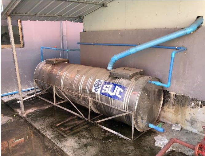
Figure 3-10 Overhead Water Storage Tank and Drinking Water Supply
