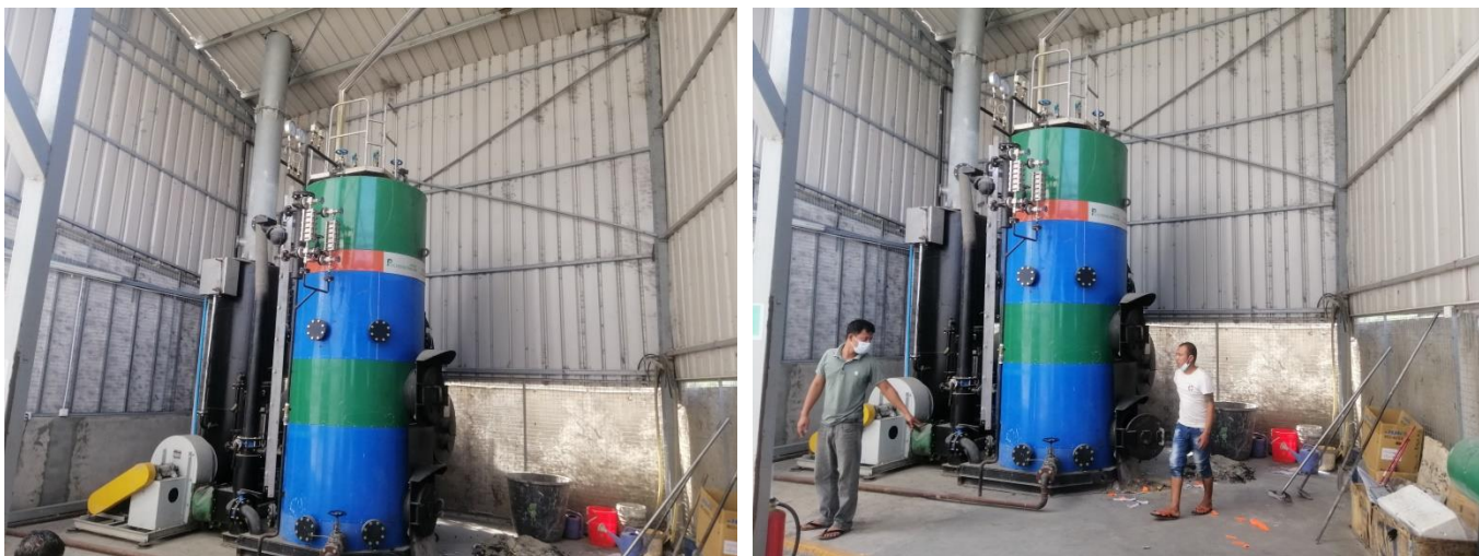
Figure 3-12 Steam Boiler Photo
