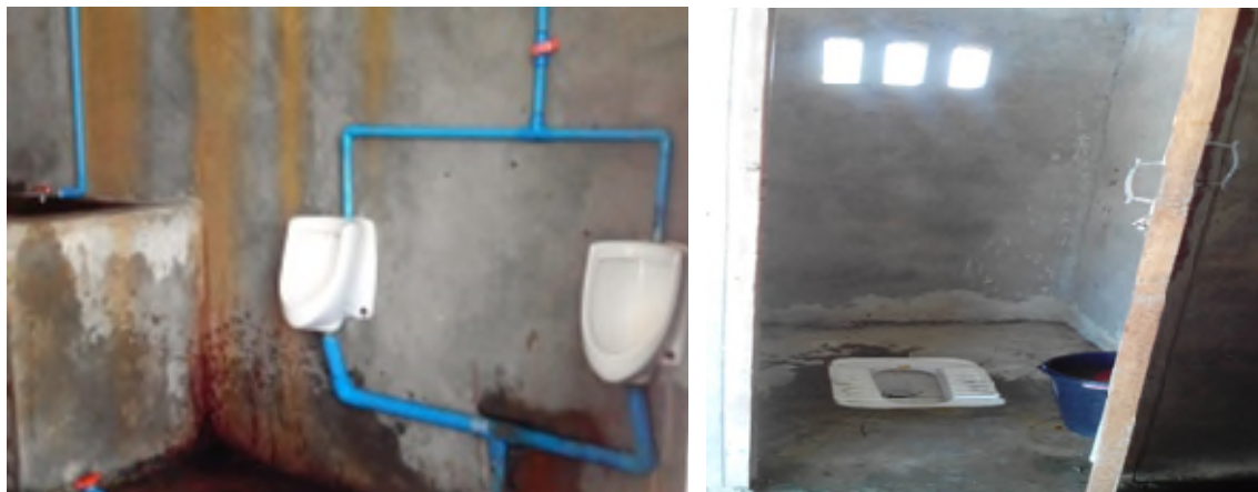
Figure 17: Toilets in Myanmar Unique Garment Factory
