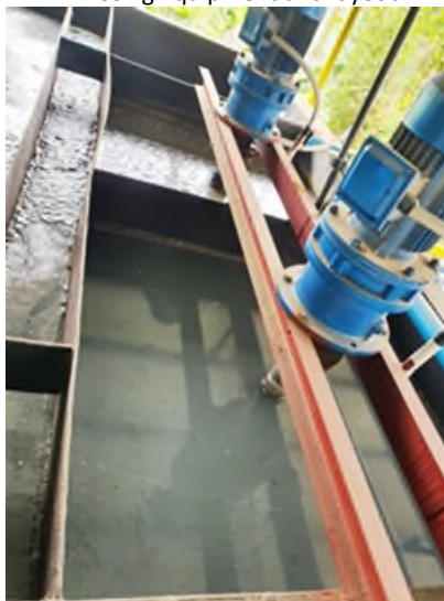
Treatment in progress
