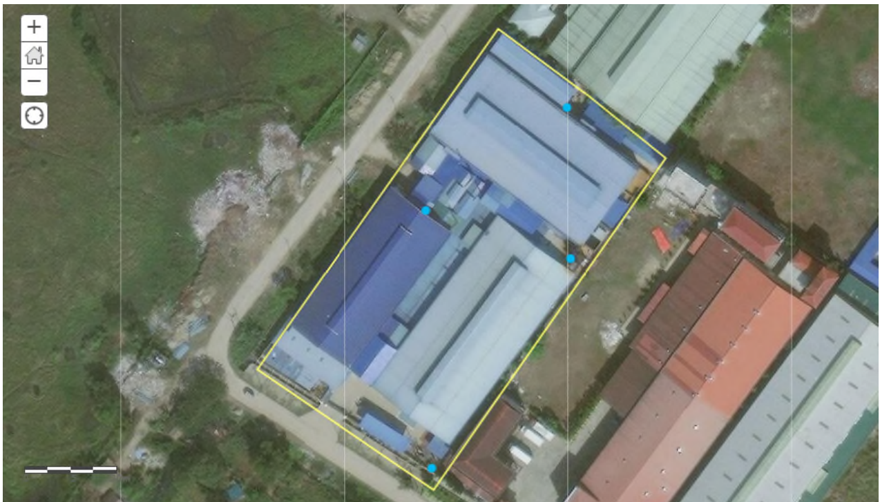
Figure 31: Tube wells location
