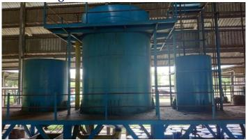
Figure 4.19 Sludge Tank, Clarification Tank and Pure Oil tank
