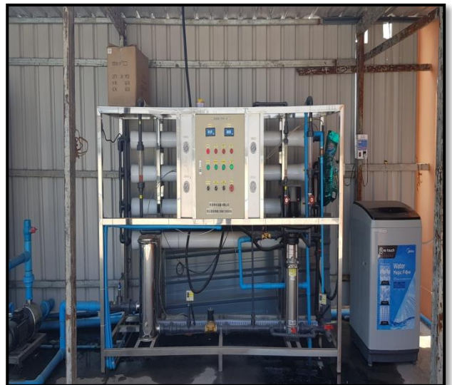
Photo 6: Water Supply and R.O Treatment
