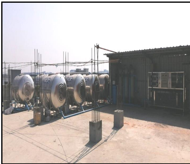
Photo 6: Water Supply and R.O Treatment
