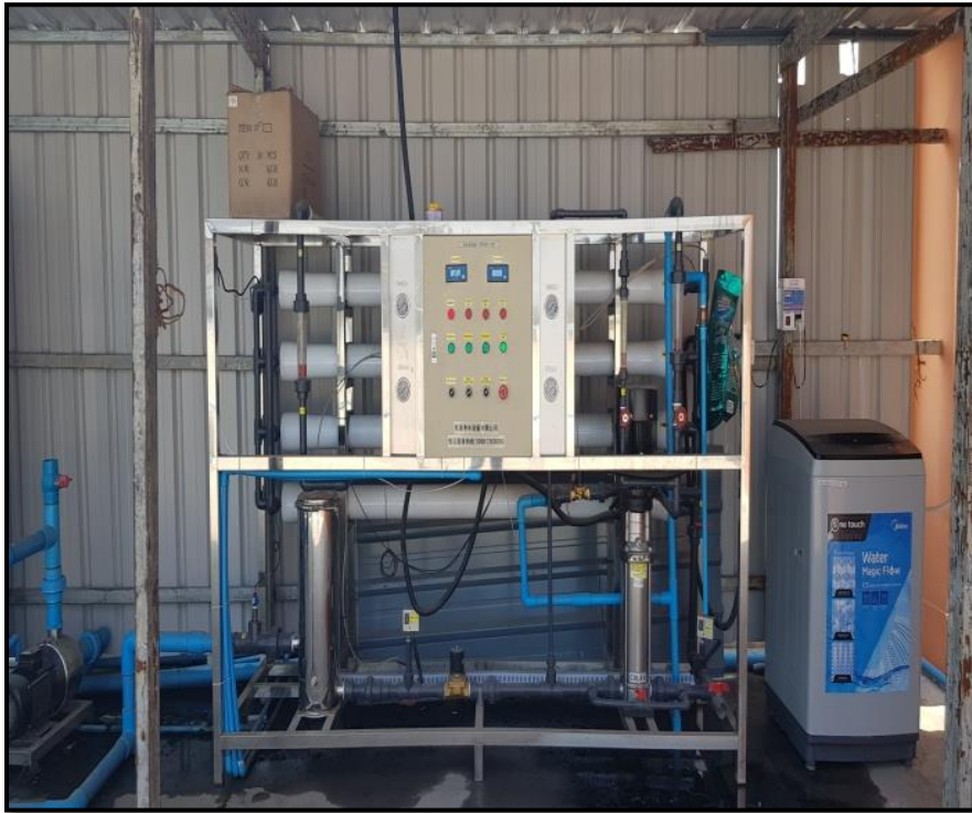
Figure 8: Mingcheng (Myanmar) RO Water Treatment Plant on site
