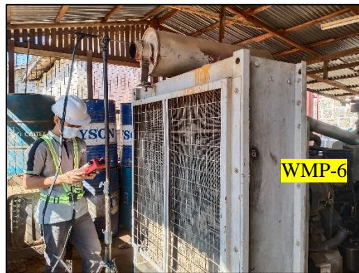
Figure 1.7 Generator Stack Measuring
