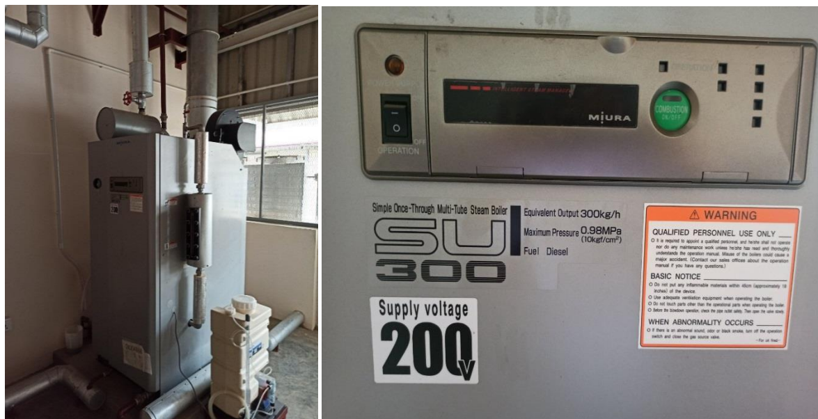
Figure 3.6 Photo of Diesel Boiler
