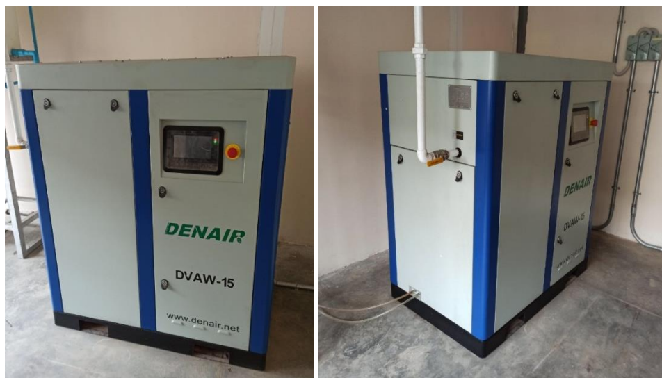
Figure 3.7 Photo of Air Compressor
