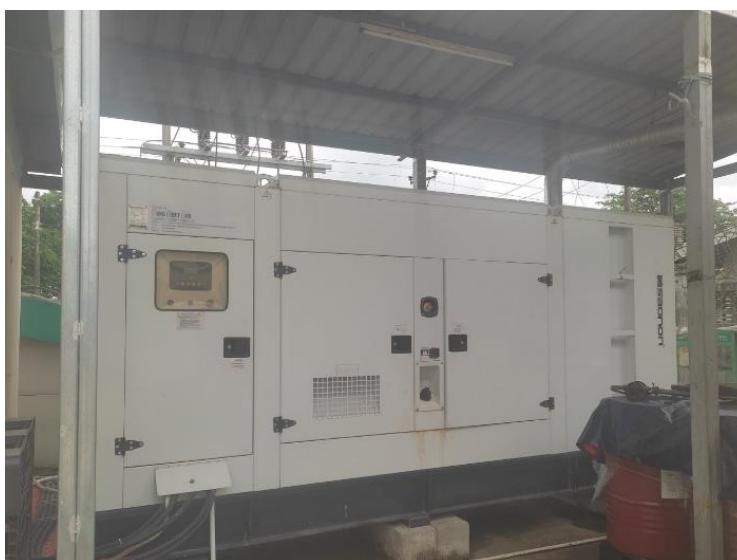
Figure 3.11 Photo of Diesel Generator (275 kVA)
