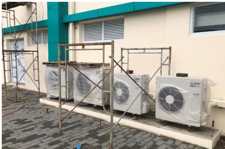
Figure 3.19 Photo of Air Conditioning System
