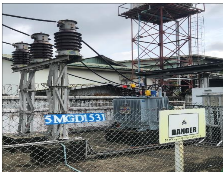
Figure 3.10 Photo of 315 kVA Transformer
