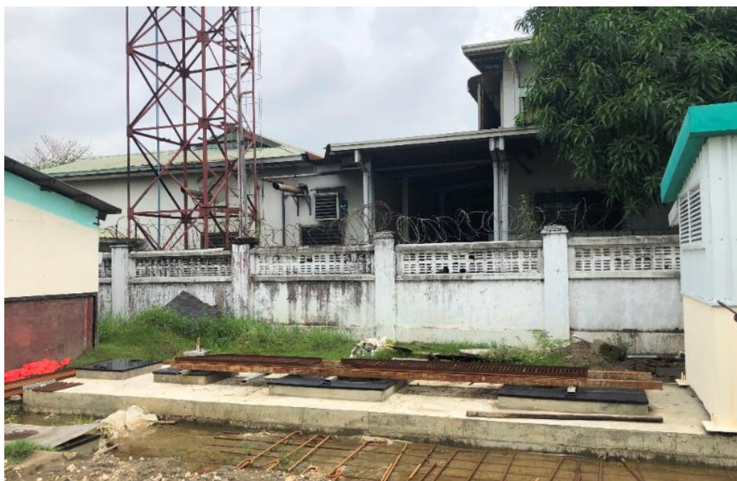
Figure 3.14 Photos of Installed WWTP
