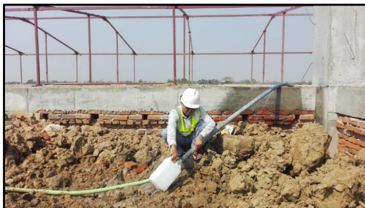
Figure 4-7 Photo of Taking Ground Water Sample from 4-inches Tube Well in the Project Site
