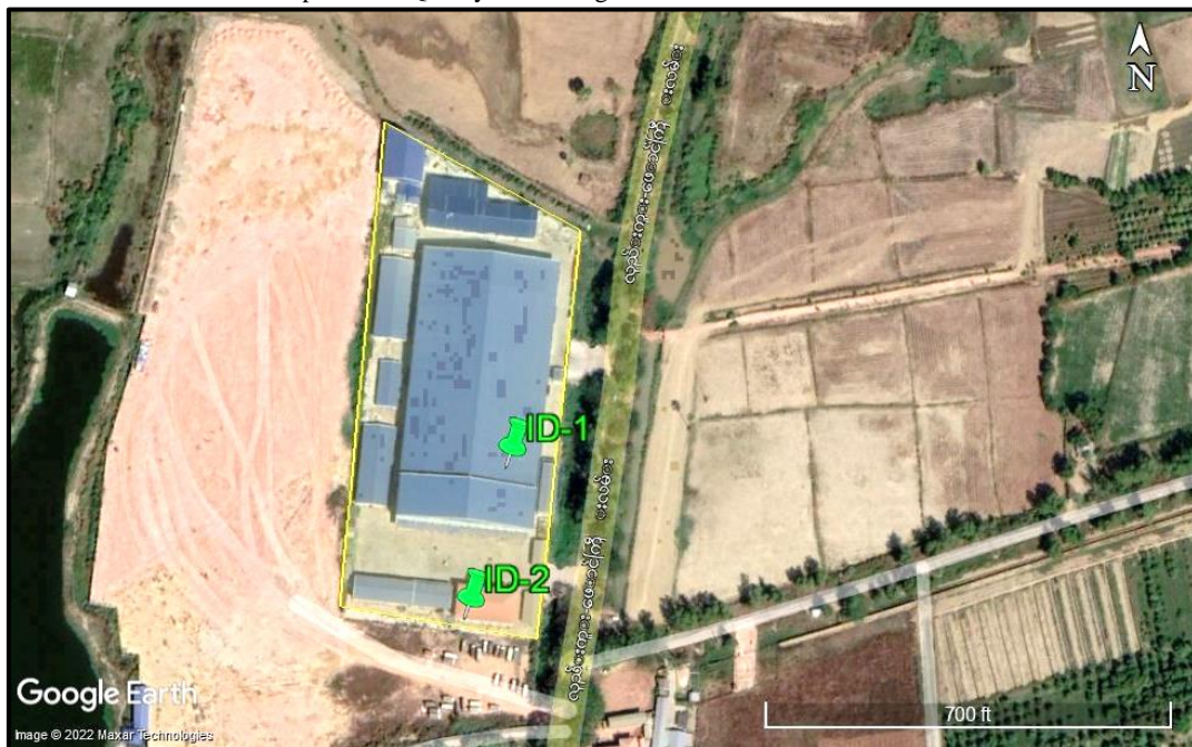
Figure 4-14 Locations of Workplace (Indoor) Noise Levels Measurement
