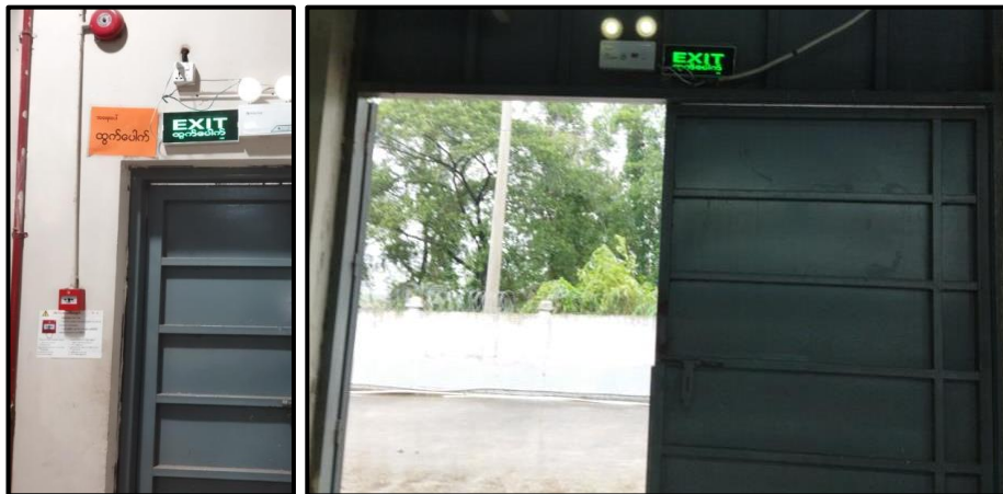
Figure 9-1 Emergency Exits and Fire Alarms
