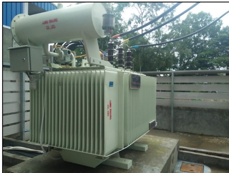
Figure 2-14 Transformer at the DMM Factory
