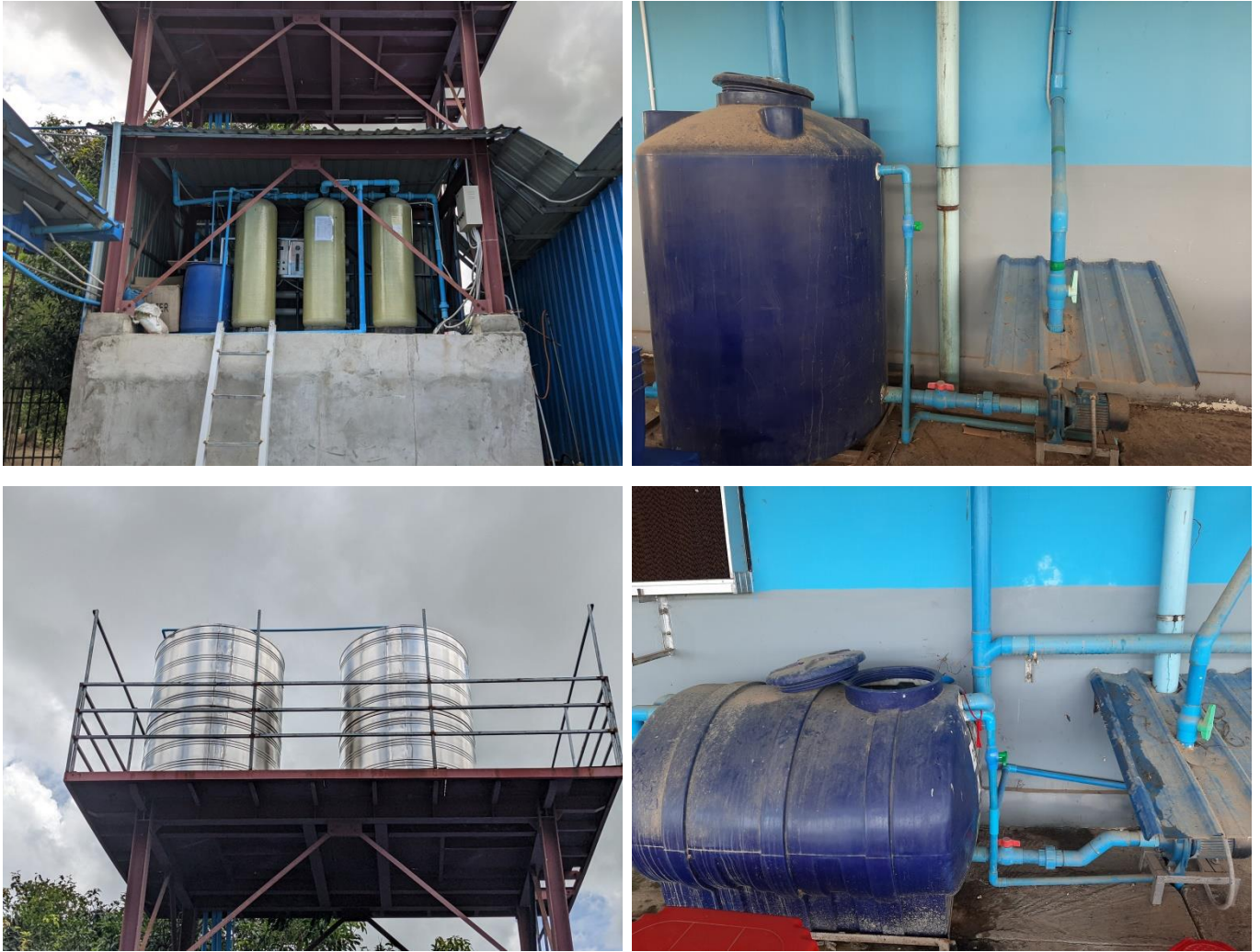
Figure 3-8 Water storage tank and drinking water supply
