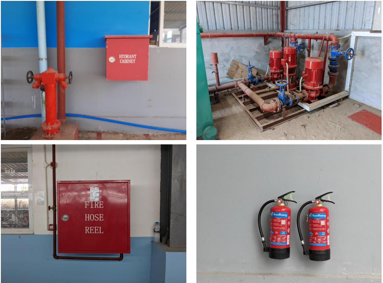
Figure 3-13 Emergency safety and fire management
