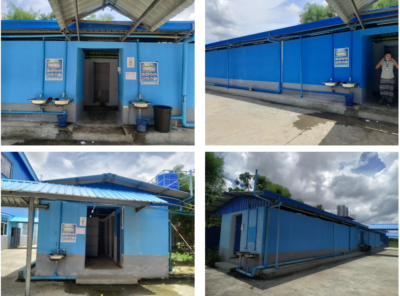
Figure 3-15 Toilet Facilities Photos
