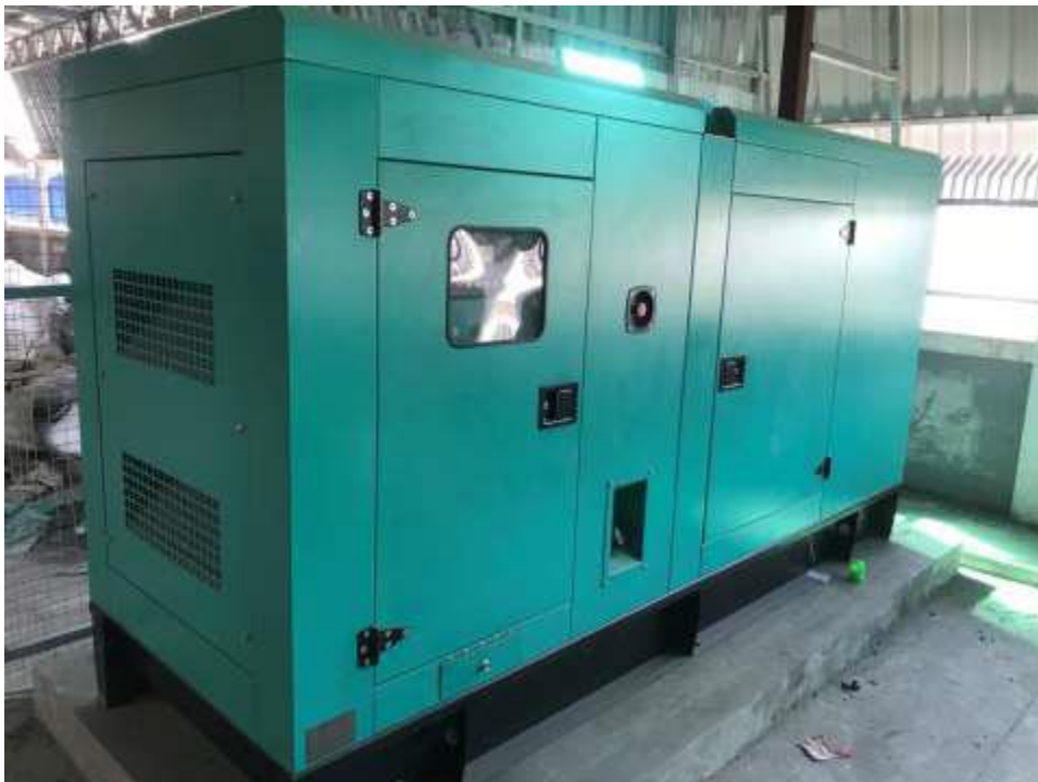
Figure 9. Noise Recovery 450 KVA diesel generator is installed
