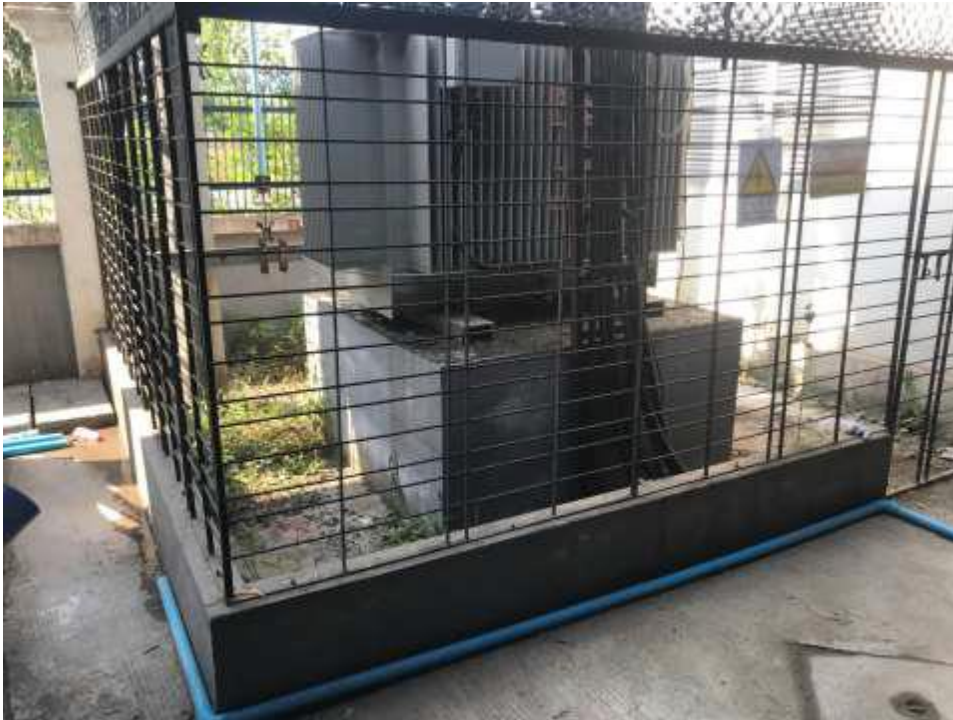
Figure 8. 1000 kVA transformers Installed
