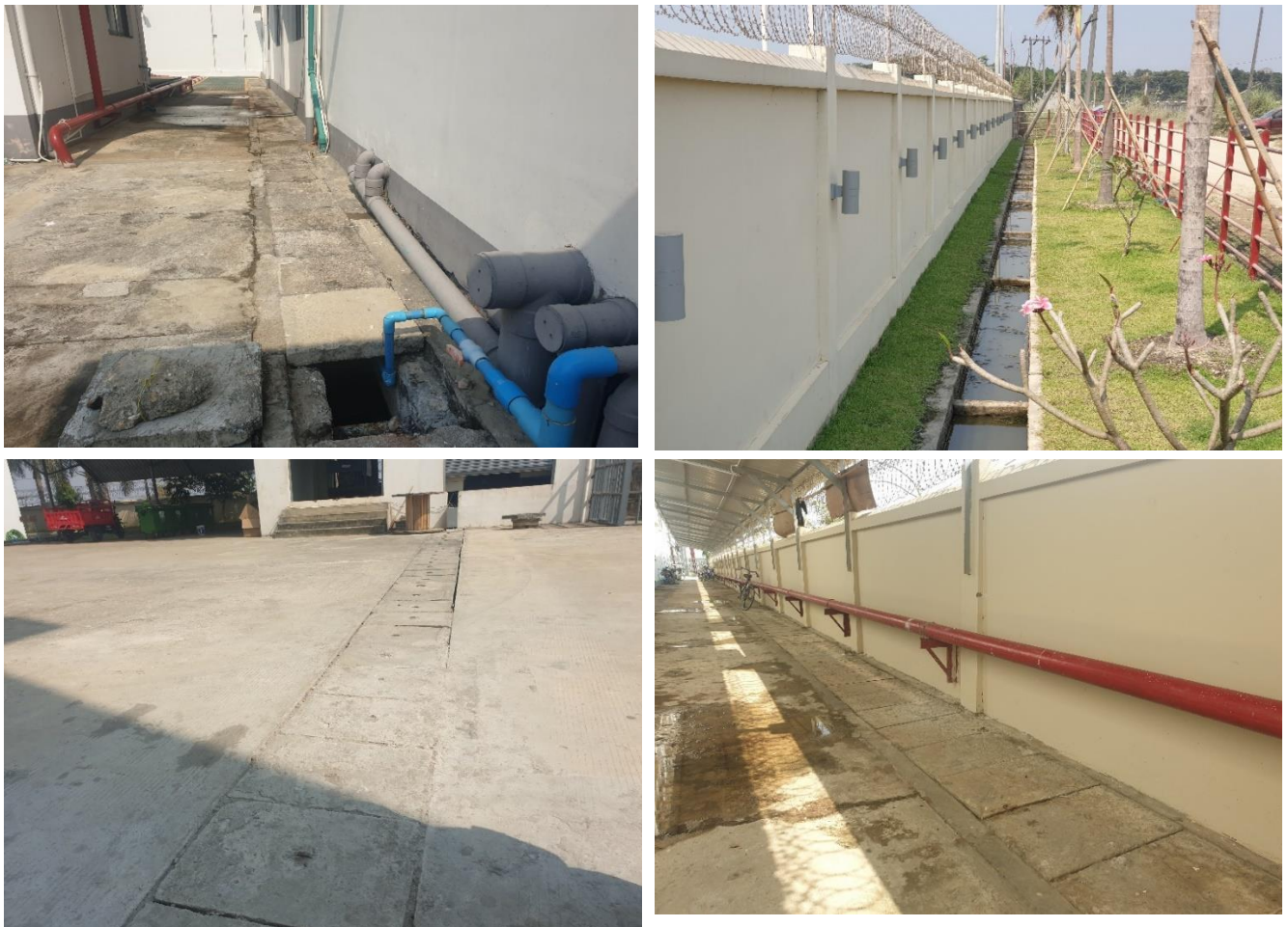
Figure 3-13 Drainage and Toilet Facility
