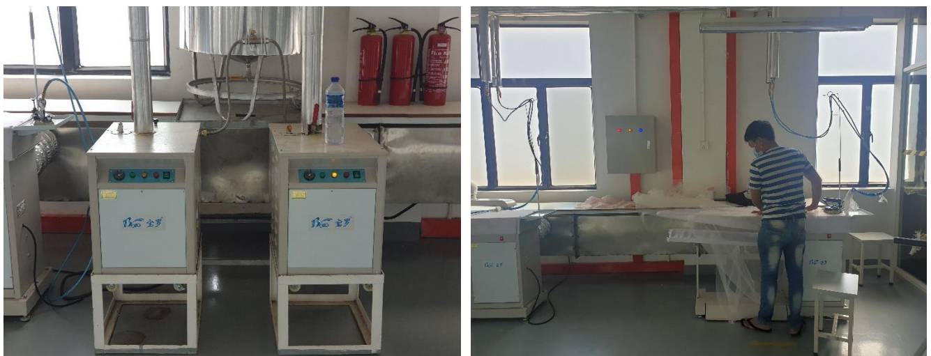
Figure 3-11 Electronic Steam Boiler
