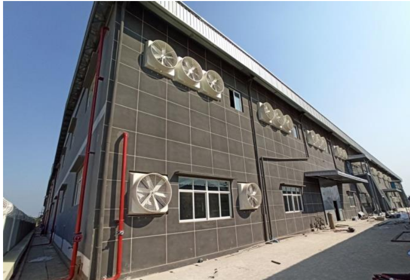
Figure 20. Exhaust Fan are Installed for Ventilation
