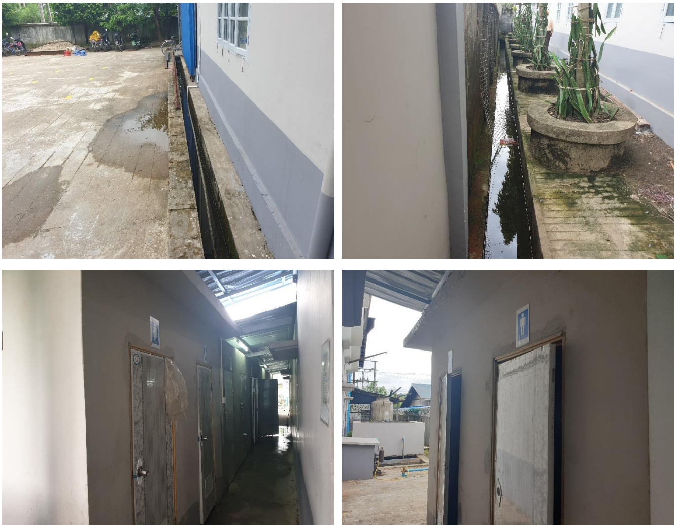
Figure 5-3 Drainage and Septic tank in project area
