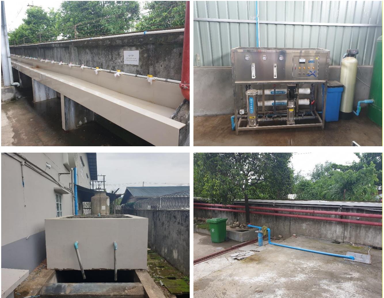
Figure 3-8 Water supply system photo
