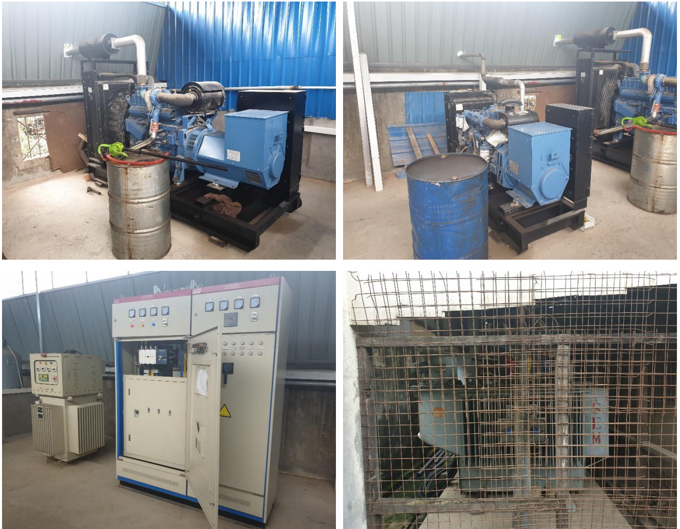
Figure 3-9 Electricity Facilities at JIN SEN MYANMAR COMPANY LIMITED
