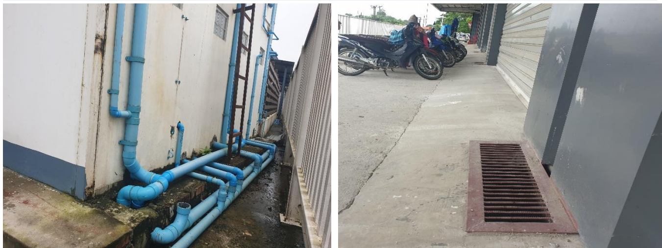
Figure 3-18 Water Drainage System
