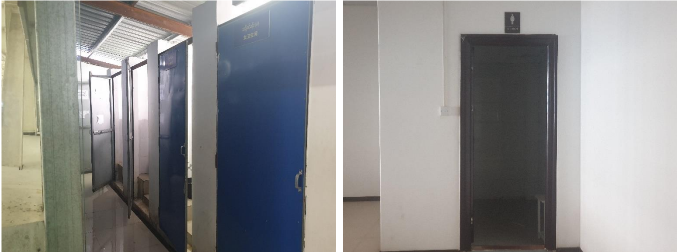
Figure 3-14 Toilet Facility Photo
