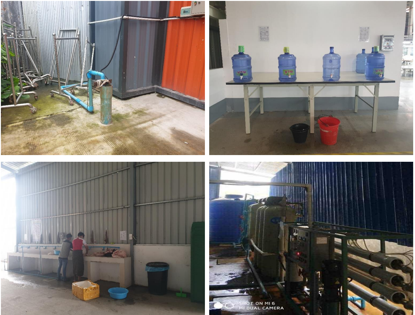
Figure 3-6 Water Supply System Photos
