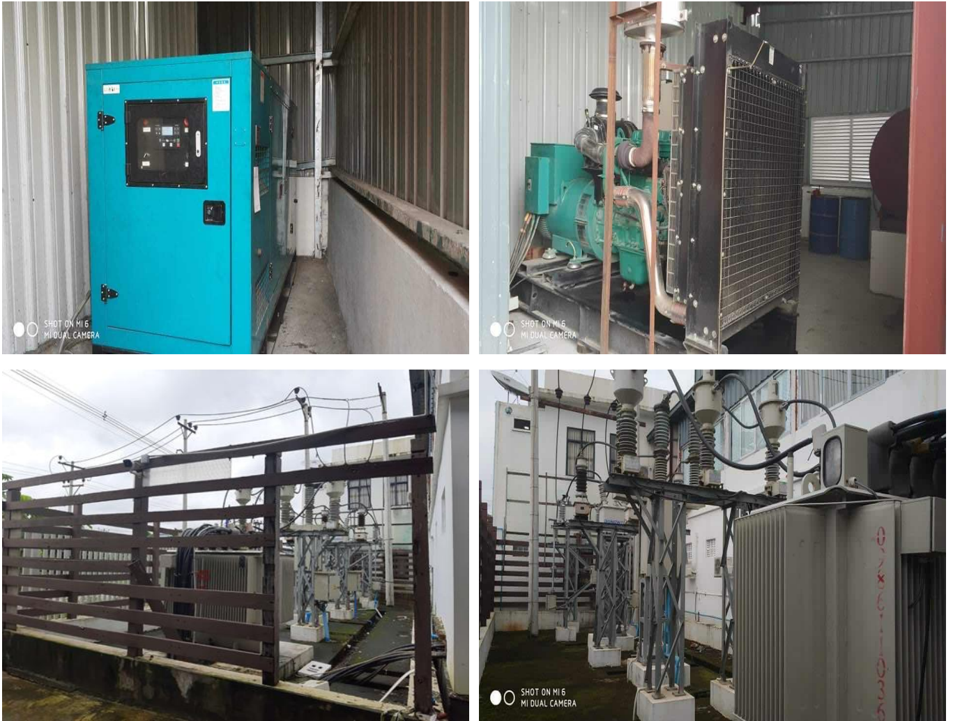
Figure 3-7 Electricity Facilities at Xinda Home Textile (Myanmar) Company Limited
