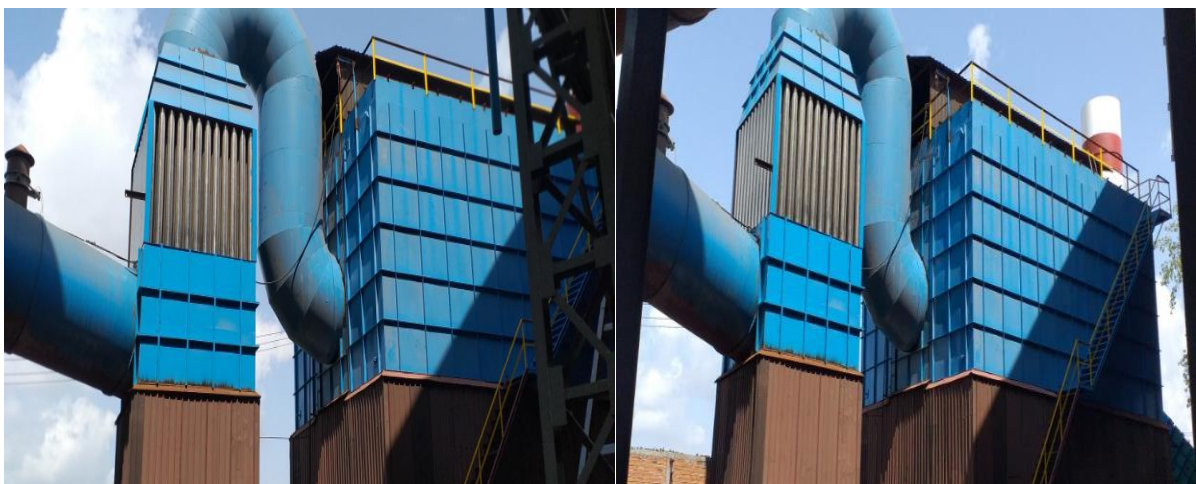
Figure 1.13 Iron Powder Fume Dust Collecting Building
