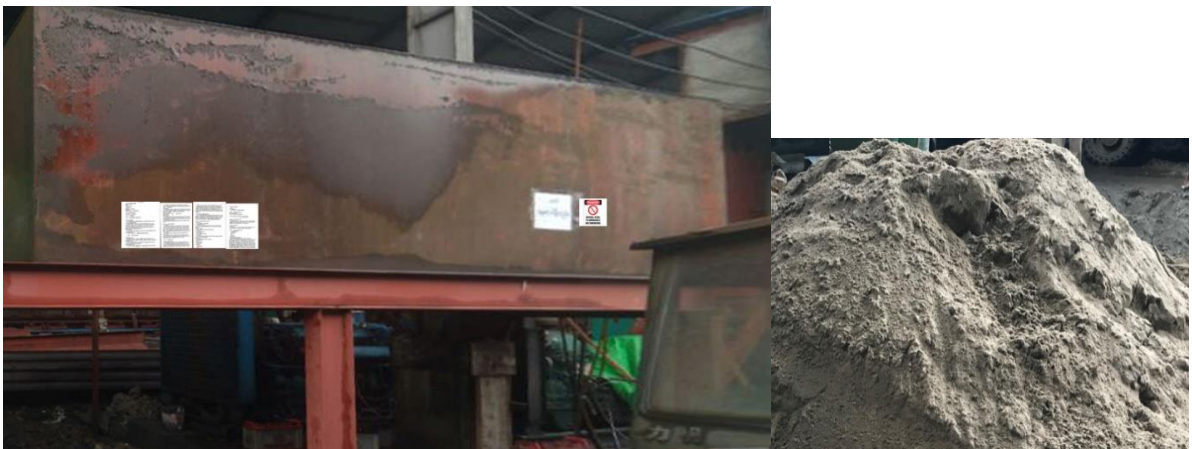
Figure 1.10 Diesel Storage Tank Post with MSDS and No Smoking Sign and Keeping Sand
