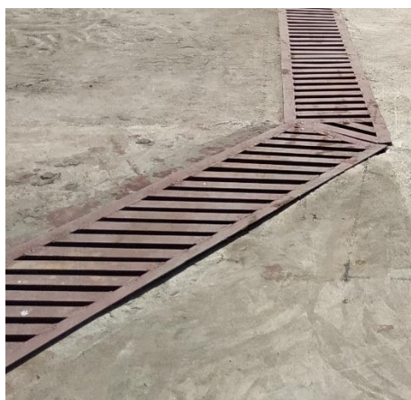
Figure 5.44 Internal Drainage
