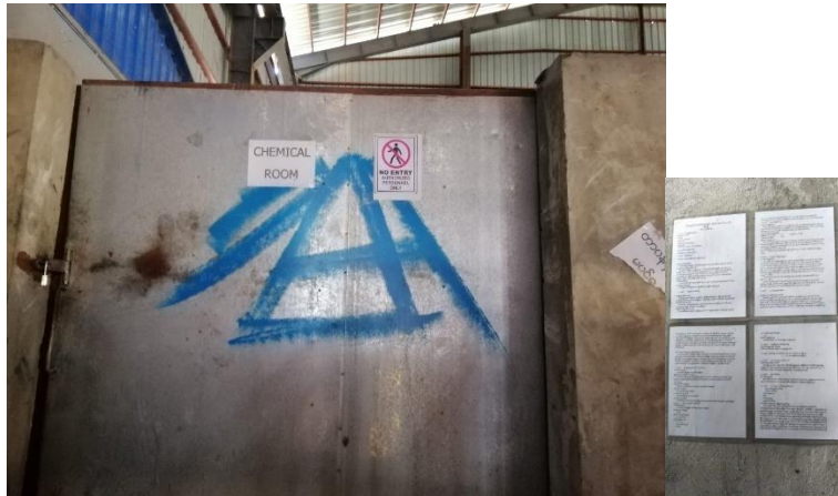
Figure 7.7 Hazardous Storage Area with MSDS, Prevent Unauthorized Individuals from Entering and Danger Sign.
