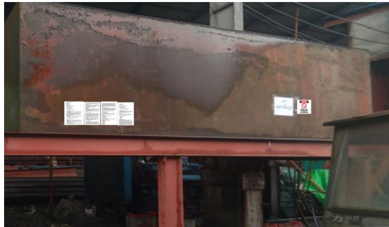
Figure 7.8 Diesel Storage Tank Post with MSDS and No Smoking Sign
