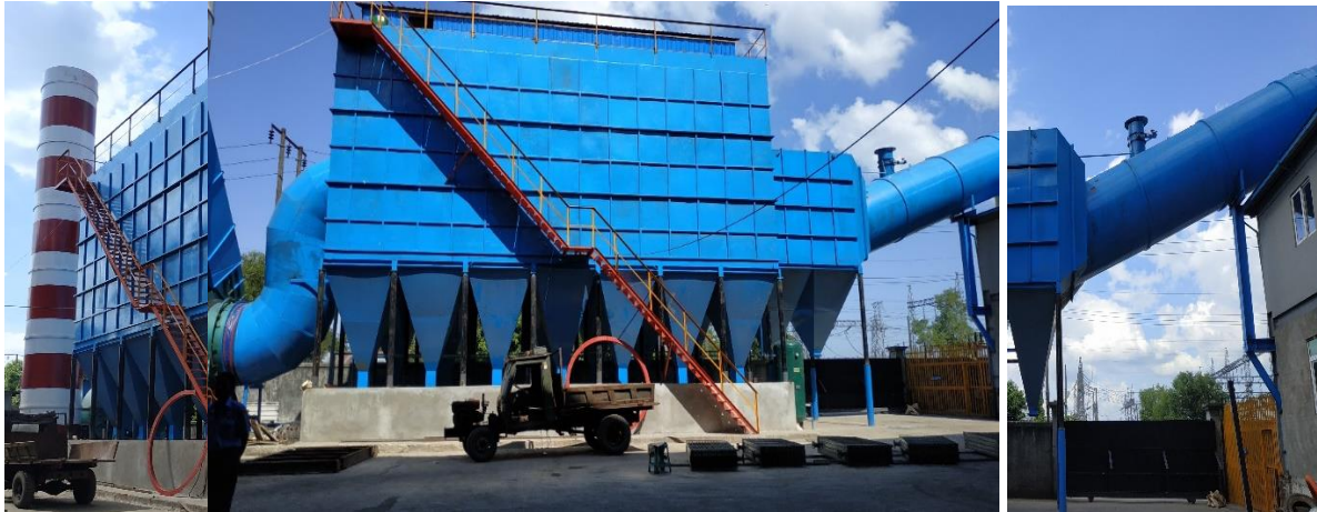
Figure 5.42 Dust Collecting Building
