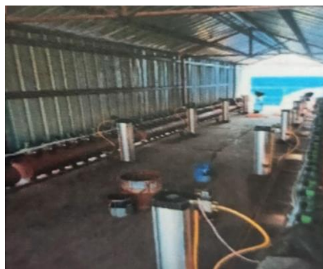
Figure 5.43 Dust Collecting System
