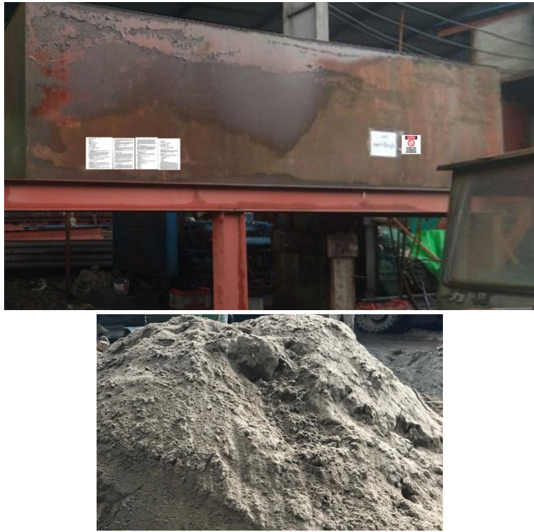
Figure 5.34 Diesel Storage Tank Post with MSDS and No Smoking Sign and Keeping Sand
