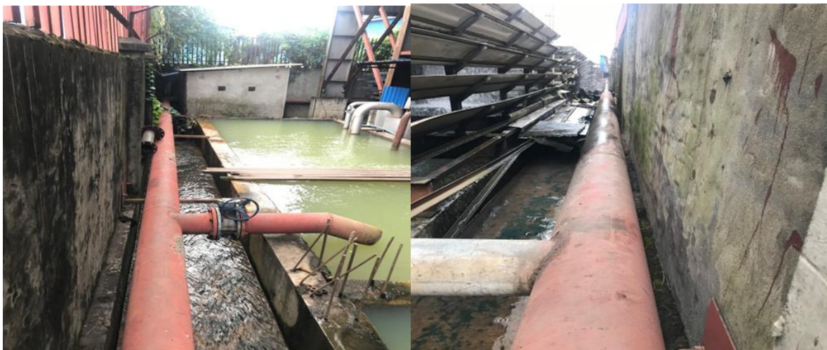
Figure 5.40 Photo Water Storage and Pipe and Water Recycle System
