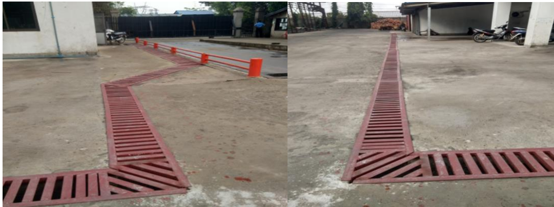
Figure 7.1 Internal Drainage of the Factory
