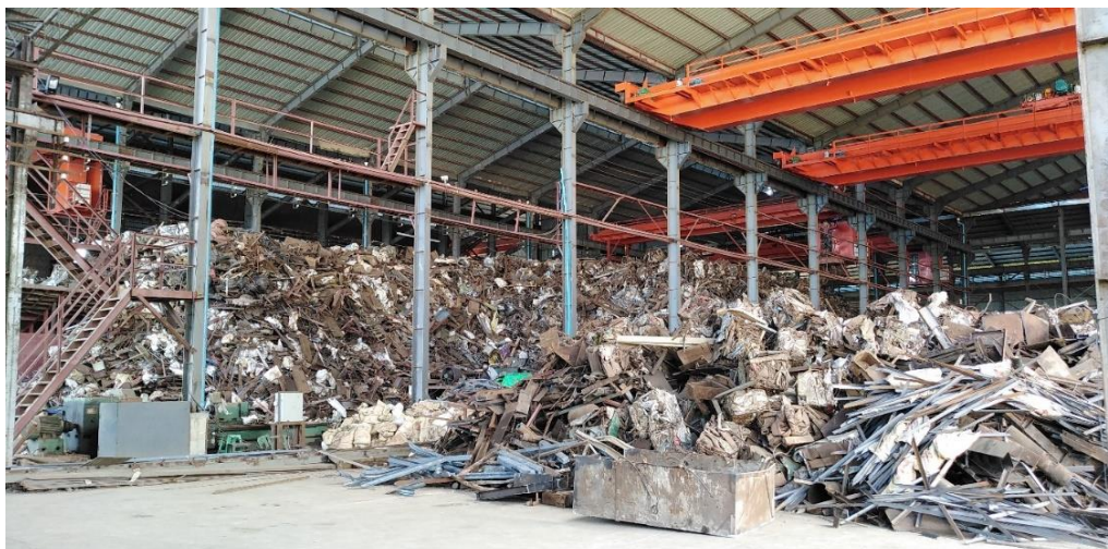
Figure 5.11 Photo of Iron Scraps and Storage Area with Roof and Concrete Floor
