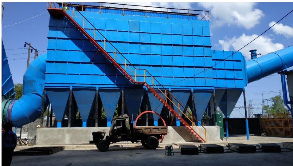
Figure 5.10 Dust Collecting Building
