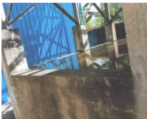
Ground Tank 4.91 x 2.8 x 0.98 m
