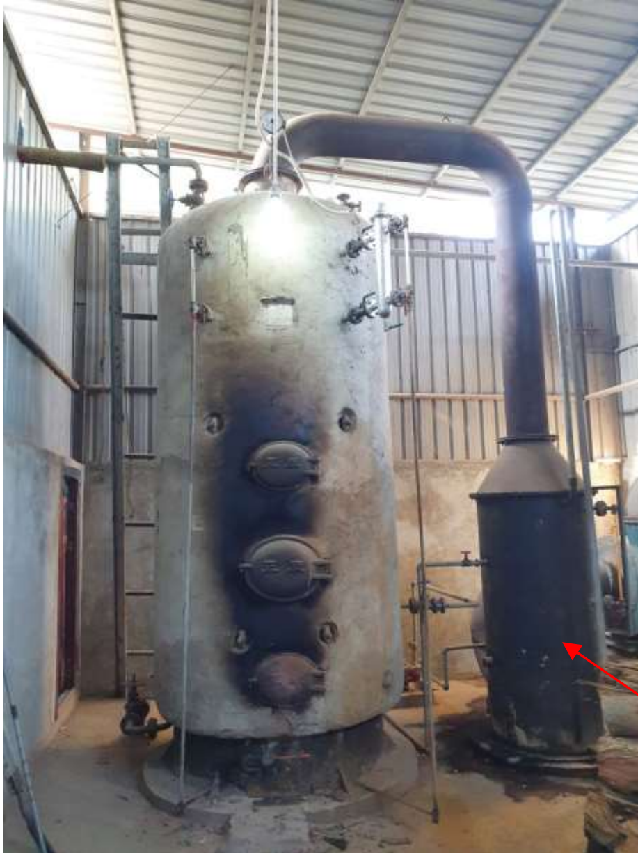
Dust / Gas Collector
