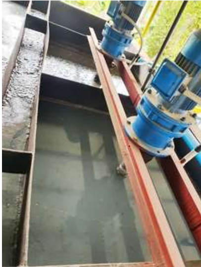
Treatment in progress
