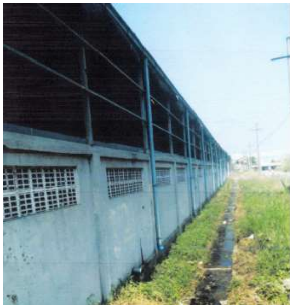
Figure 32: Public Drain beside the factory
