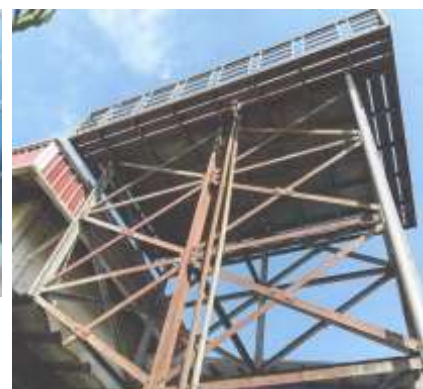
Overhead tank 4.91 x 2.8 x 2.33 m
