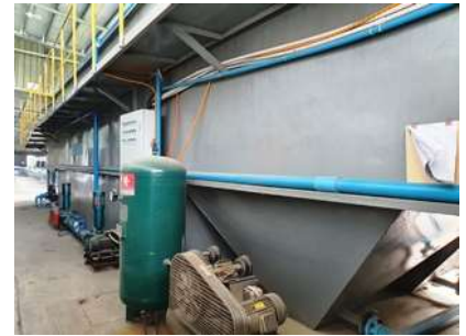
Wastewater treatment equipment
