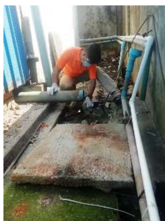
Figure 44: wastewater collection point
