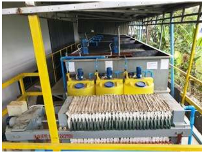
Dosing Equipment and layout
