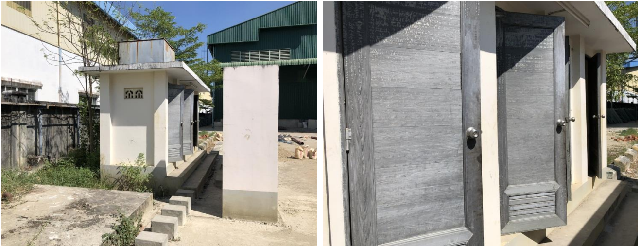
Figure 3-10 Toilet facility at RANDOO (MYANMAR) SILK CORP., LTD
