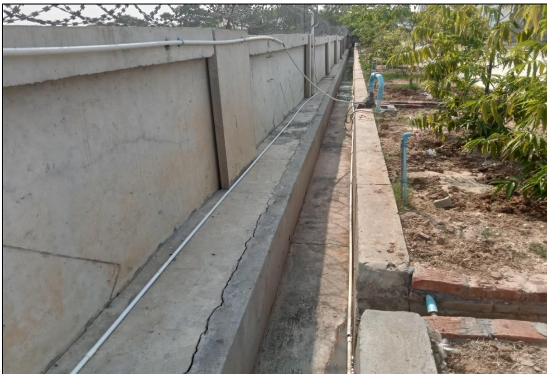
Figure 2-29 Factory Drainage Channel
