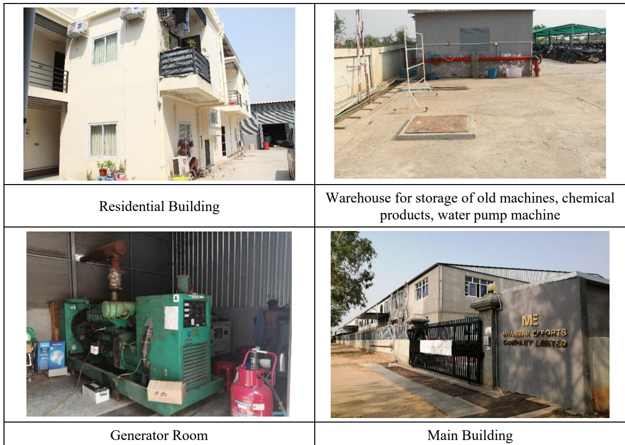
Figure 2-3 Buildings in the Project Area
