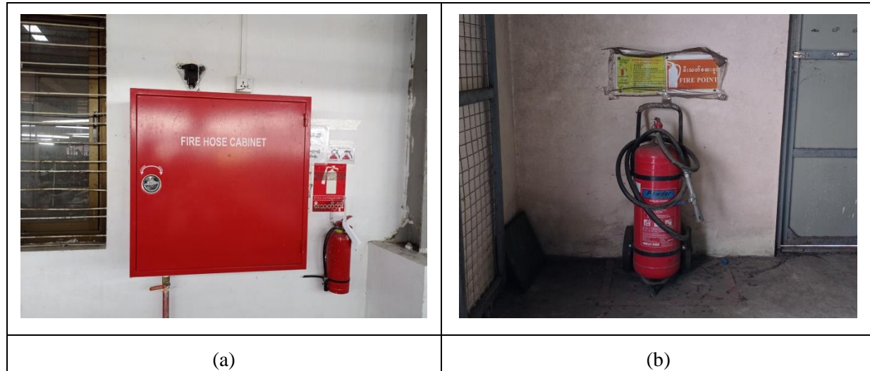
Figure 3.14 (a) Portable Fire Extinguisher and (b) Wheeled Fire Extinguished
