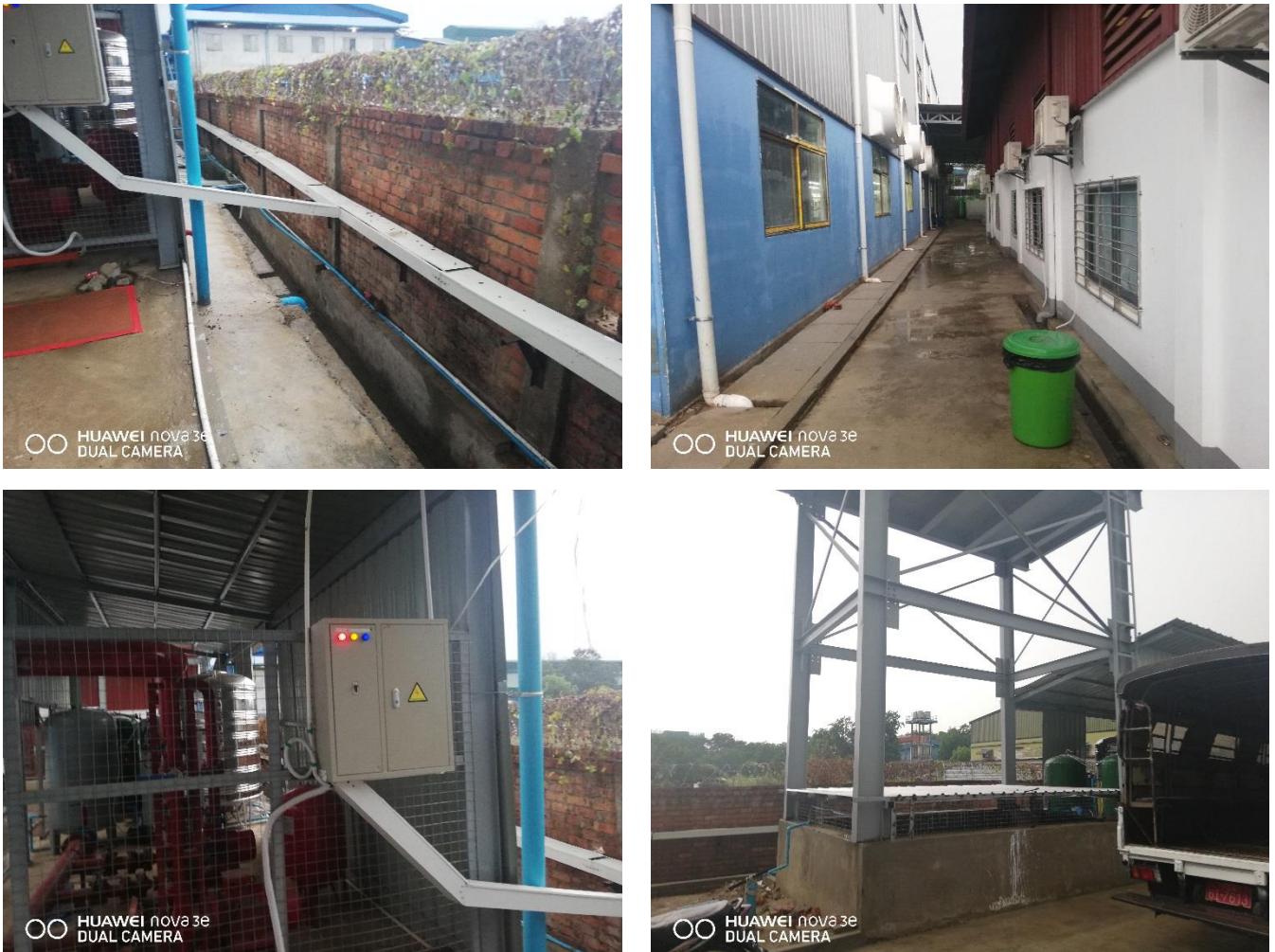
Figure 5-3 Drainage and Septic tank in project area
