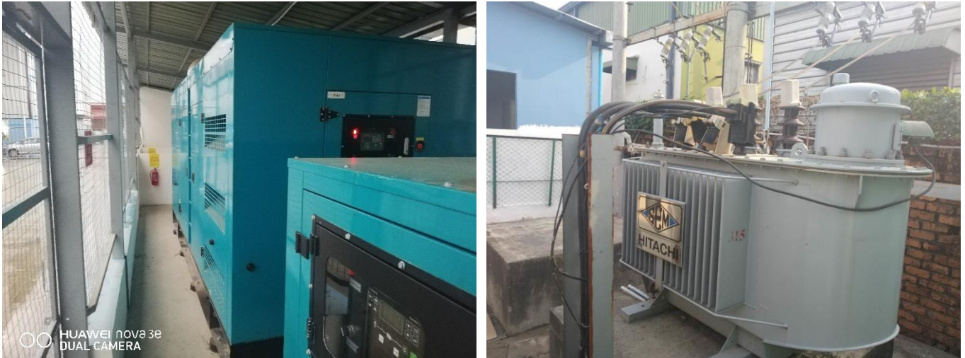
Figure 3-8 Electricity Facilities at Bo Da (Myanmar) Fashion Factory
