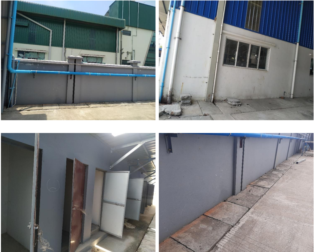
Figure 1-13 Drainage and Toilet facility
