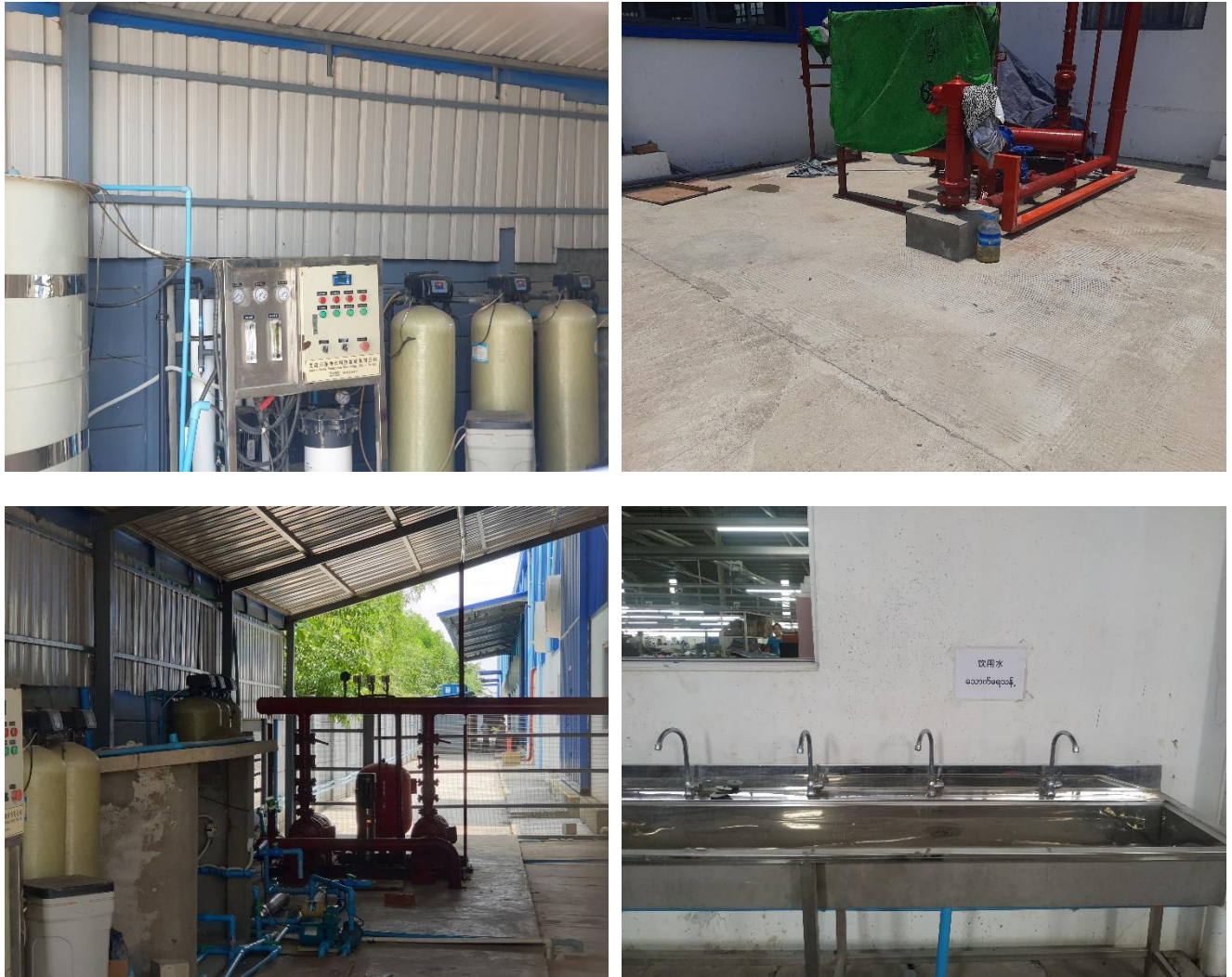
Figure 1-10 Underground water storage tank and drinking water supply
