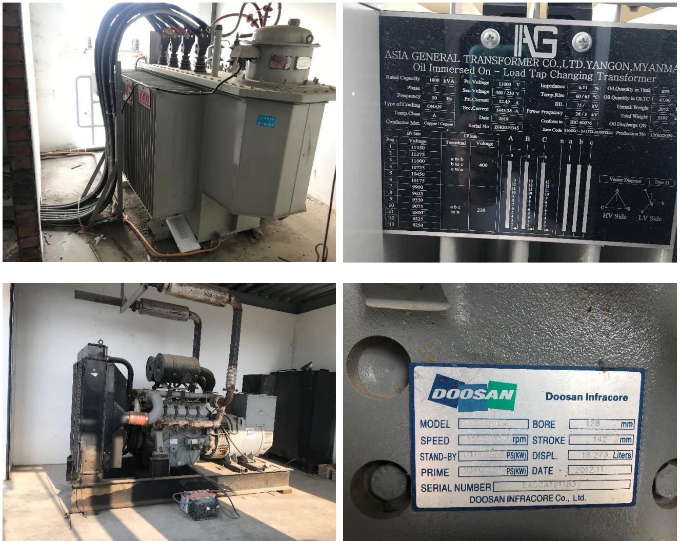
Figure 1-11 Electricity Facilities at FINELINE Factory
