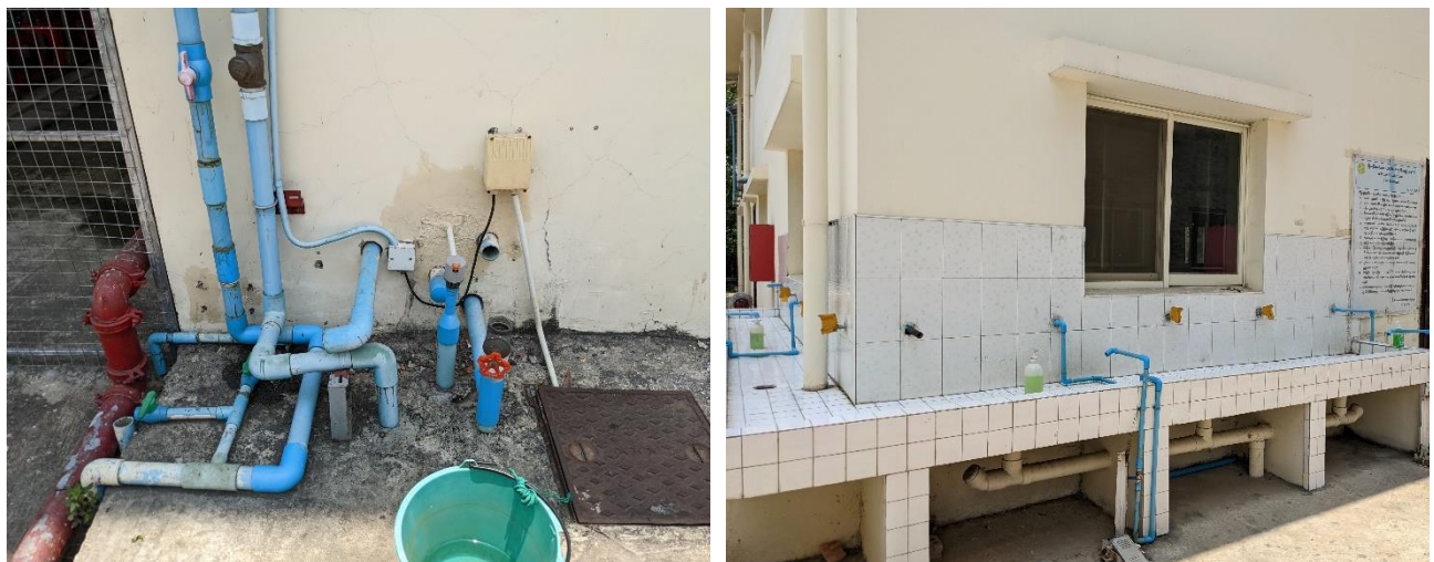
Figure 3-7 Underground water storage tank and water supply
