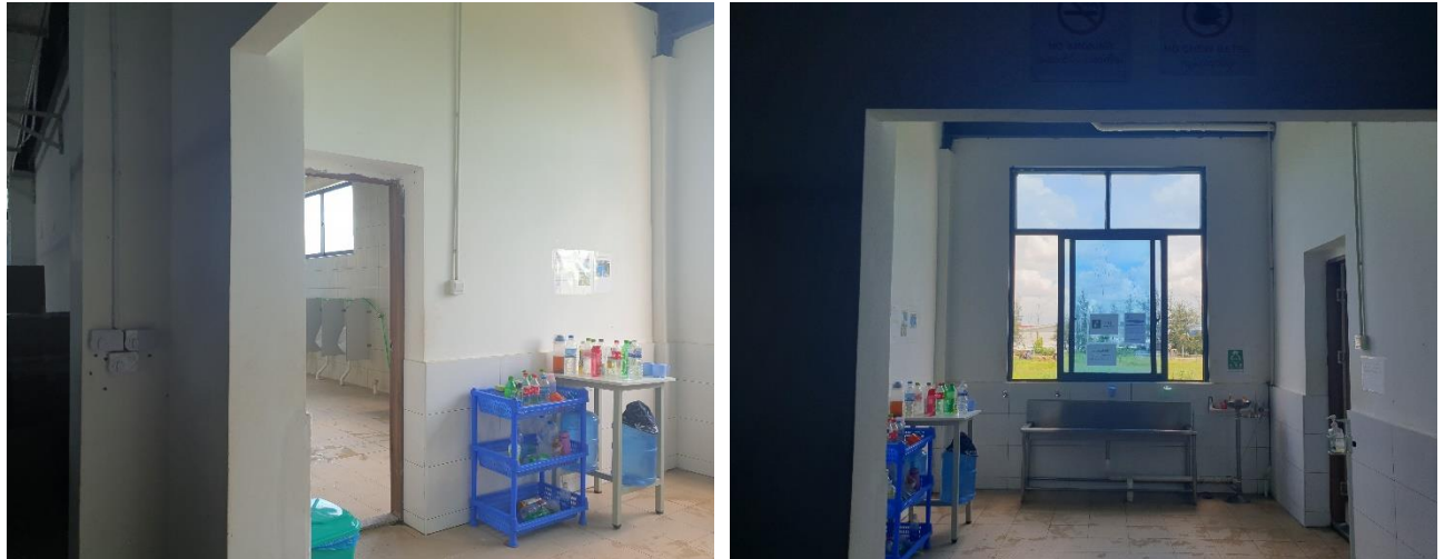
Figure 3-12 Toilet Facility in Factory
