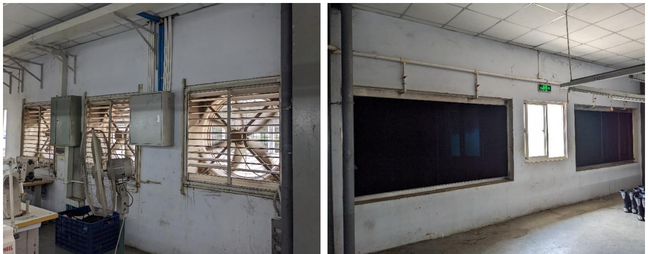
Figure 3-13 Ventilation System at factory
