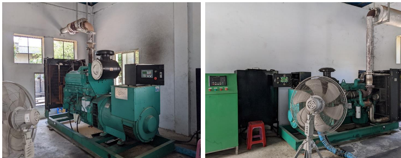
Figure 3-8 Electricity Facilities at William (Myanmar) Industrial Company Limited Factory
