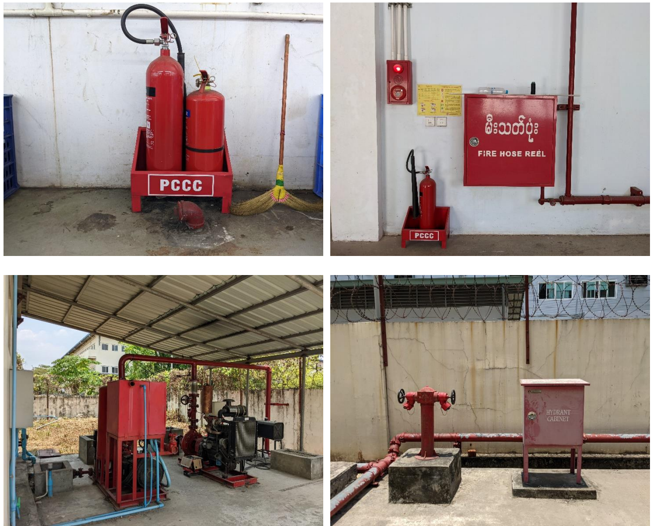
Figure 3-9 Firefighting system
