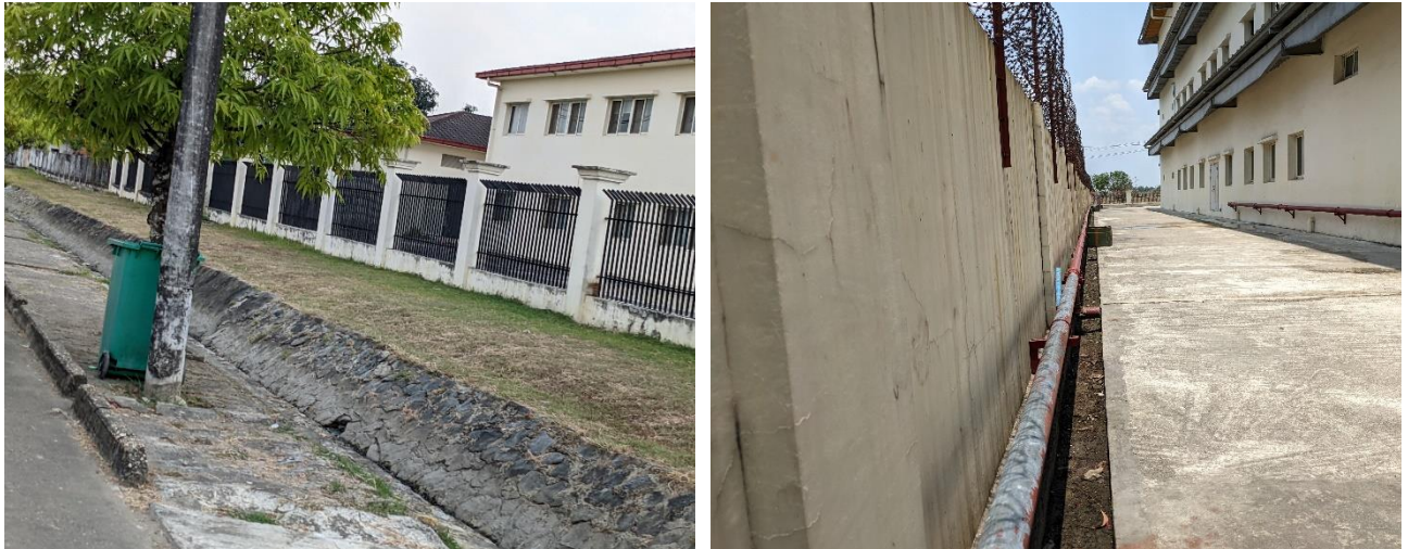
Figure 3-10 Drainage and Toilet facility
