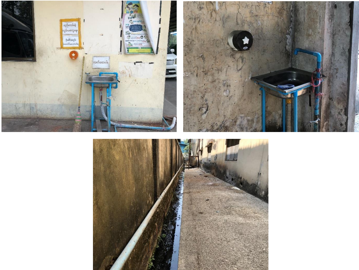
Figure 6. 9 Toilets, Washing Basins and Drainage System
