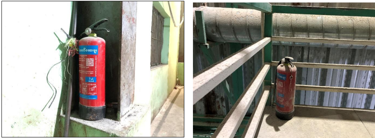
Figure 6. 6 Installed Fire Extinguishers
