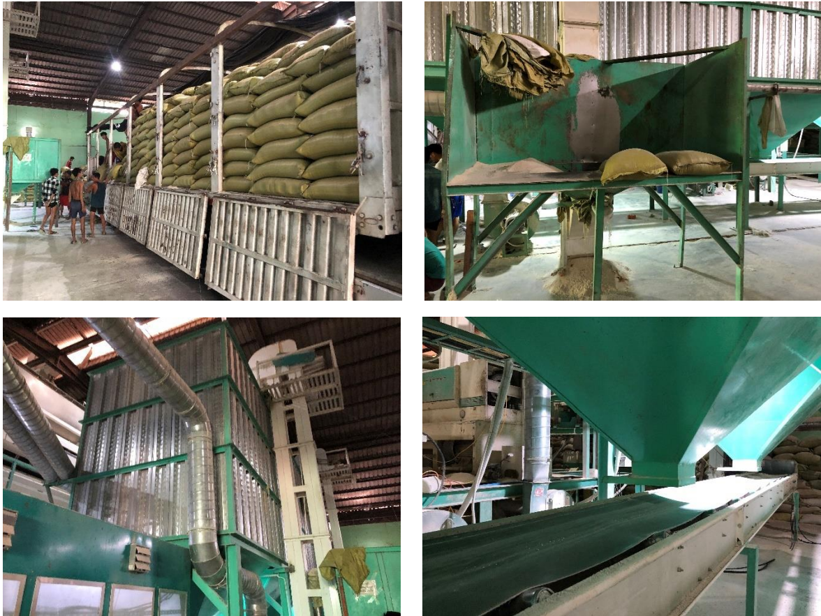
Figure 1. 7 Inlet, Raw Rice Tank and Conveyor
