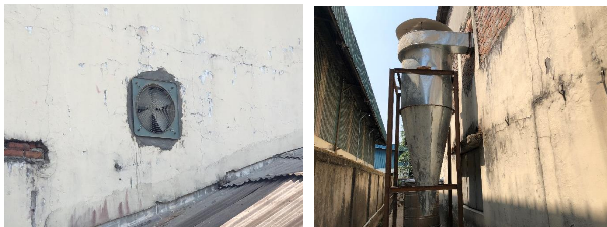
Figure 6. 3 Installed Exhaust Fans and Cyclone Dust Collector
