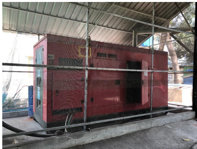
Figure 6. 4 Installed Silence-type Diesel Generator
