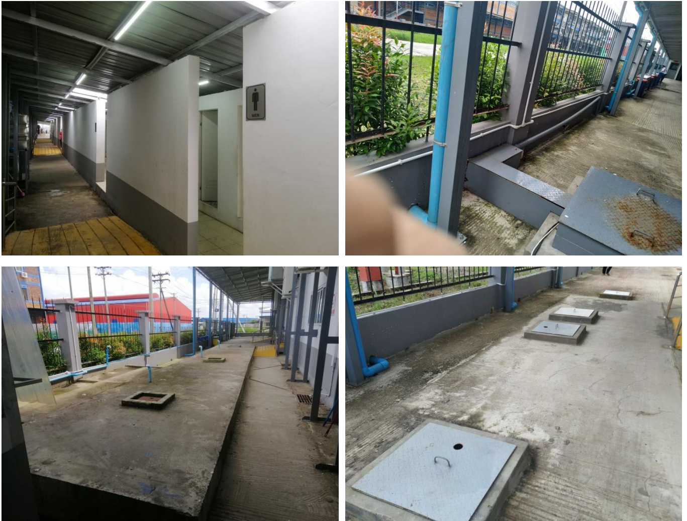
Figure 3-14 Drainage and Toilet facility
