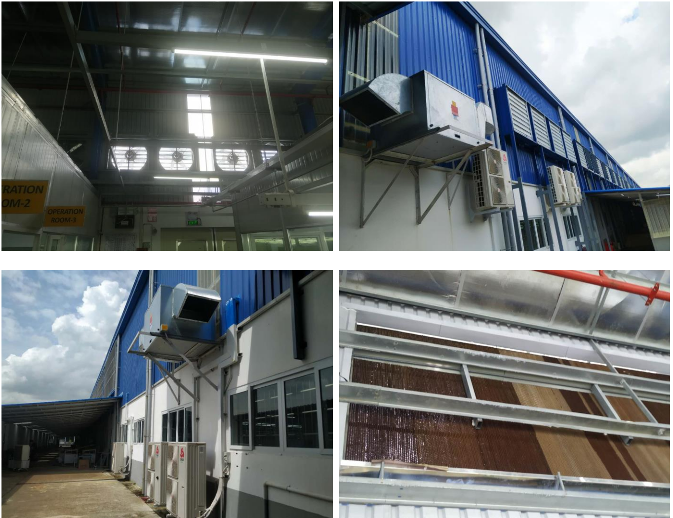
Figure 3-13 Ventilation System Photo
