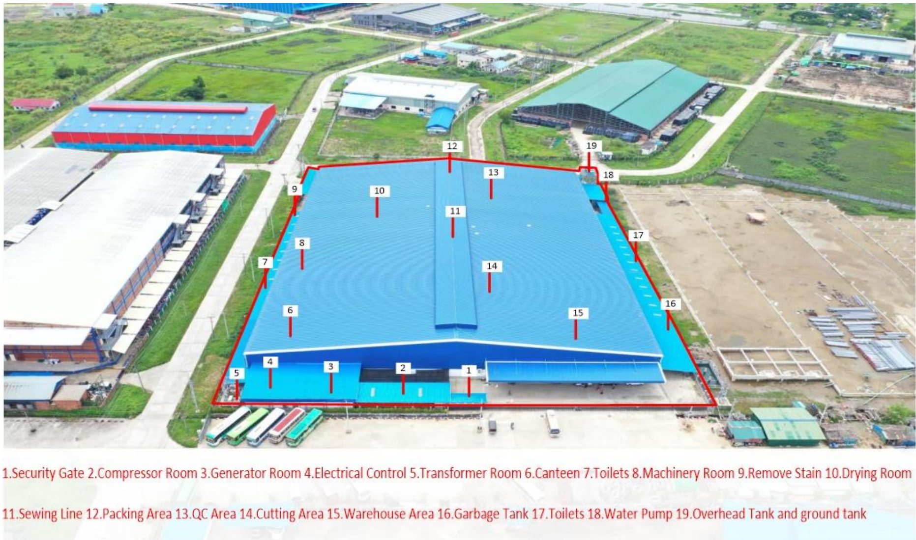
Figure 3-3 Factory Aerial Photo
