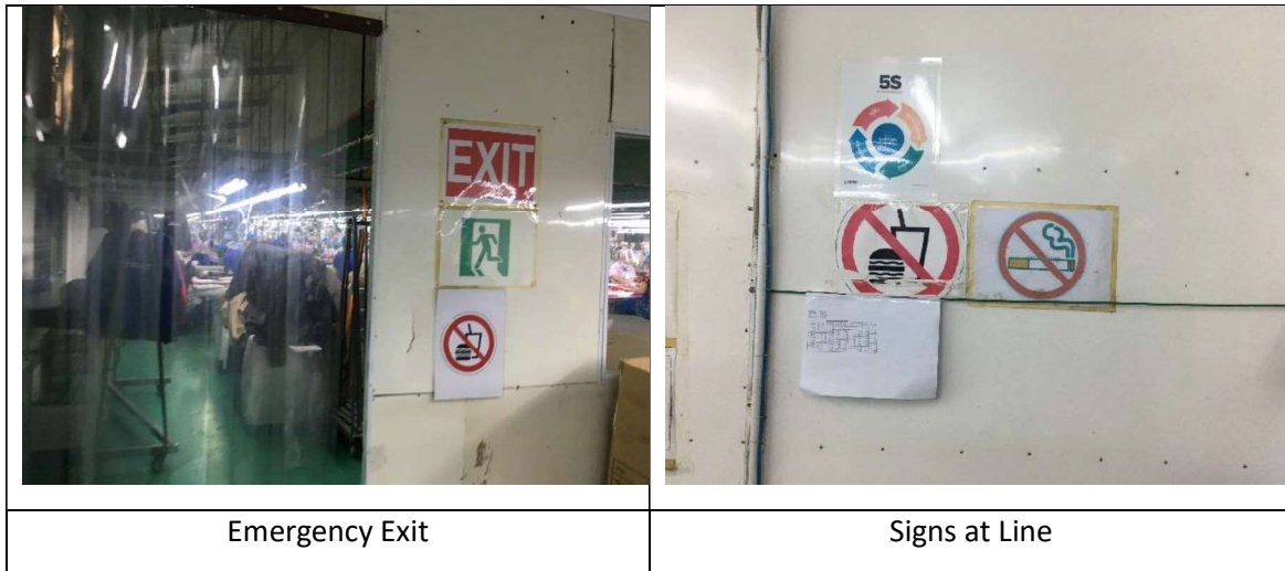
Figure 7-8 Fire-fighting and Emergency Response Facilities at THY Garment Factory
