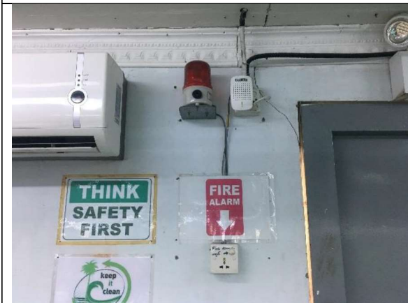
Fire Alarm at QC Room
