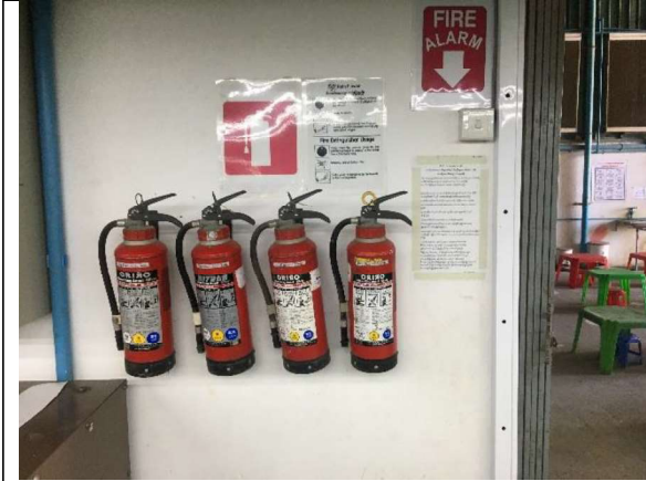
Fire Extinguisher at Cutting Room
