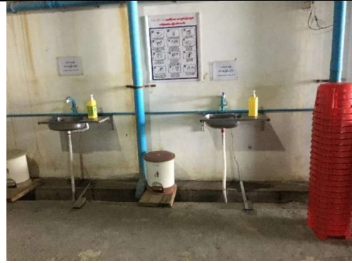
Hand Wash Basin(In Dining Room)
