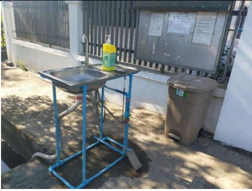
Hand Wash Basin(In front of Main Gate)
